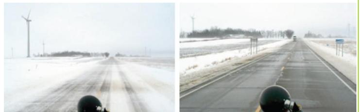
Segments of roads with LSFs (right) have better driver visibility and road surface conditions than those without (left), leading to lower road maintenance costs and fewer accidents. LSFs can also benefit the atmosphere by storing carbon dioxide and reducing emissions from snow removal operations.
