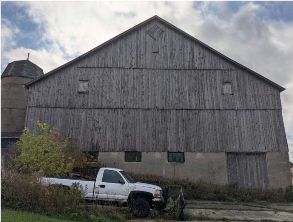
Figure 76: North elevation of large barn
