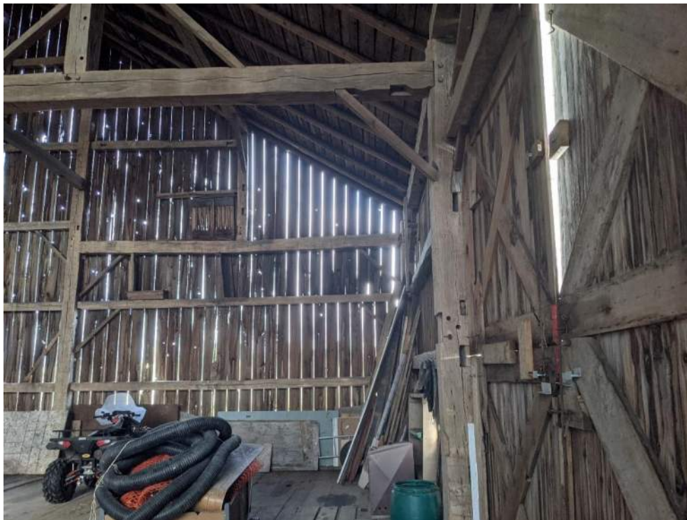
Figure 81: Interior of the large barn, note the extra mortises in the hand-hewn beams
