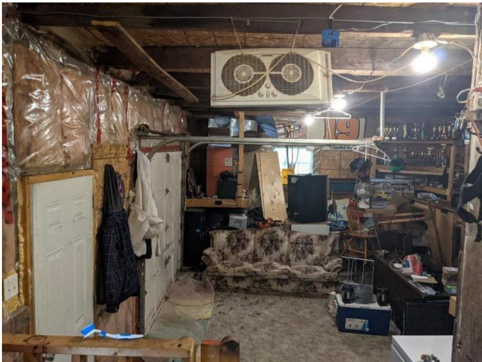
Figure 60: Interior of north addition, facing north
