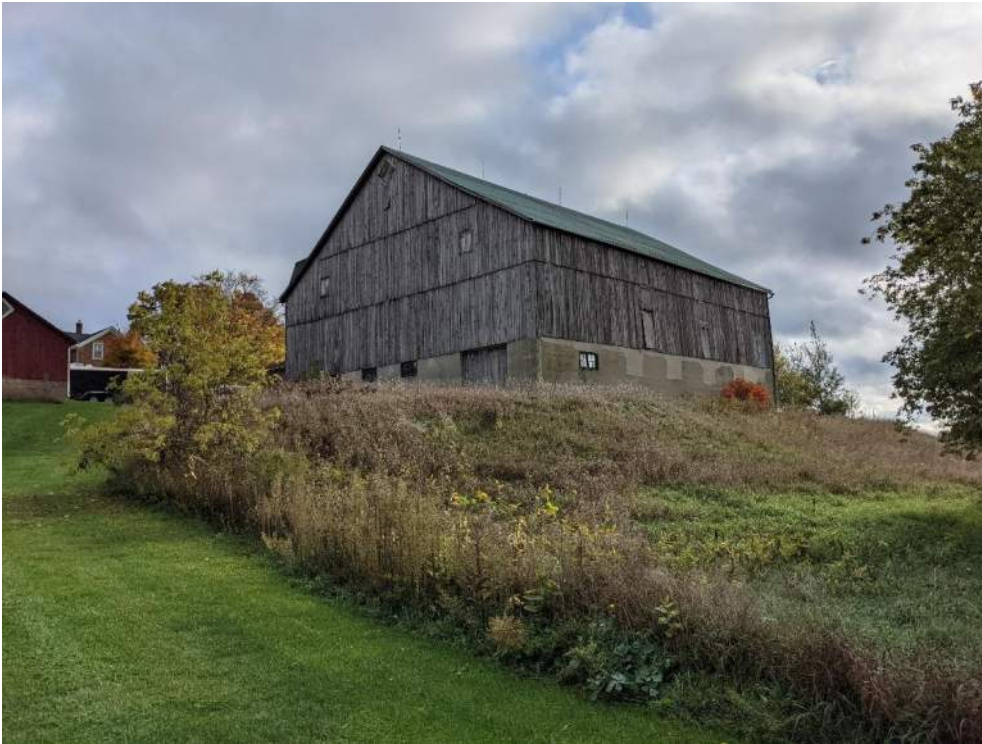
Figure 78: West and south façades of the large barn
