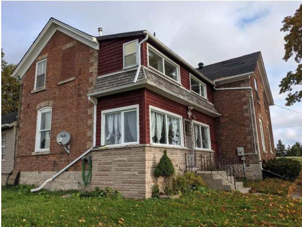
Figure 62: The south and west elevation of the south addition
