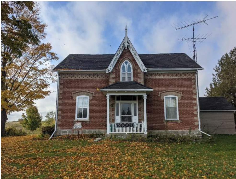
Figure 13: Front or east façade of the Farmhouse
