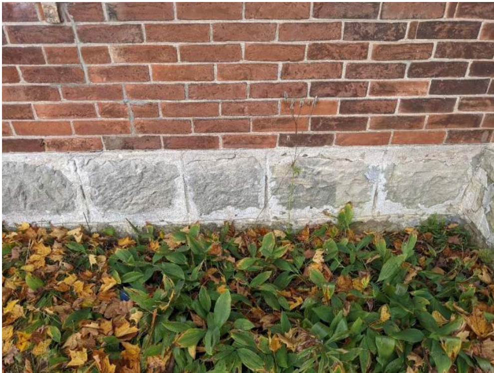
Figure 18: Tooled stone foundation and running bond brick on the east façade
