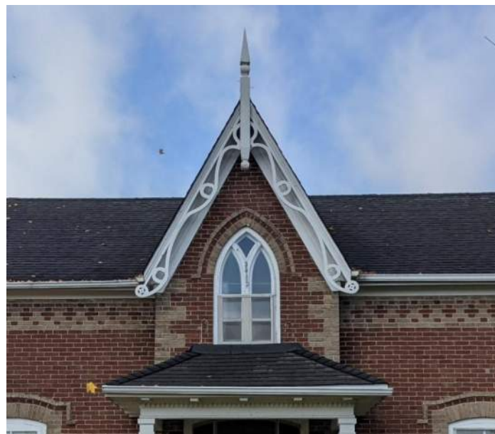
Figure 21: Gable peak on east façade
