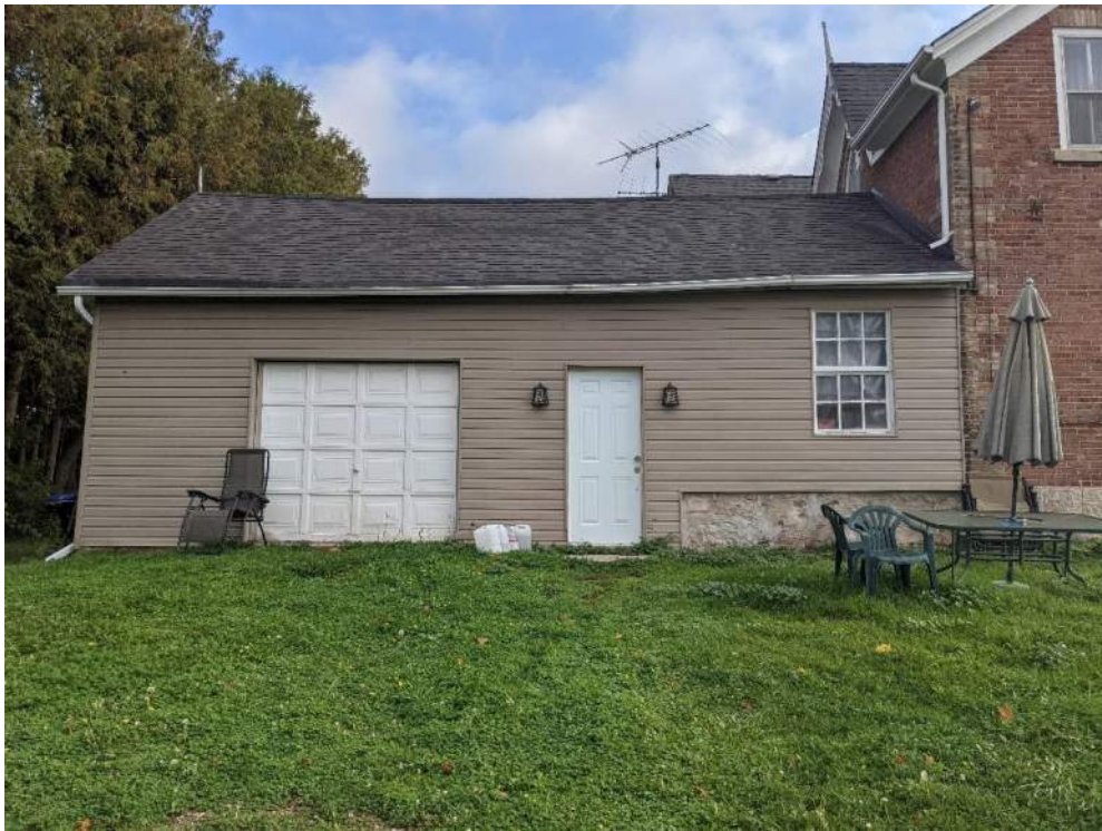
Figure 55: West elevation of the north addition
