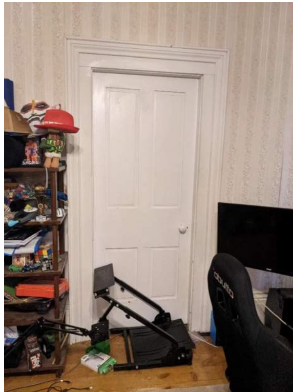
Figure 31: Four paneled door in north front room
