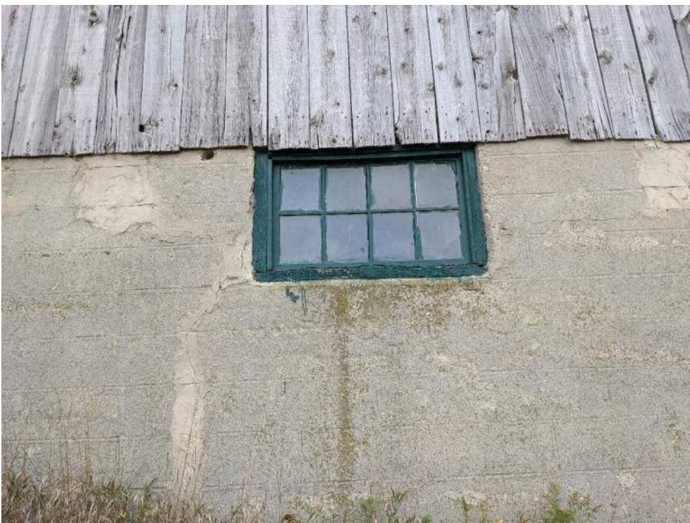
Figure 77: Typical window on the north elevation of the large barn
