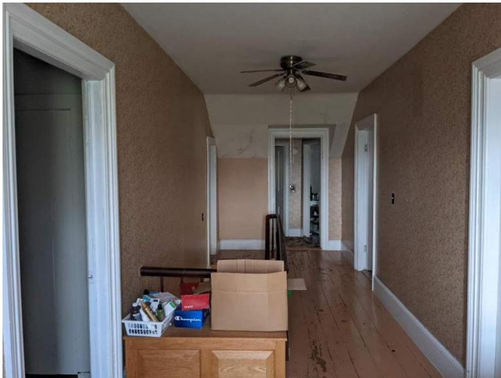
Figure 42: Second level hall landing, looking west
