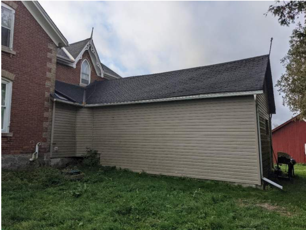
Figure 57: West elevation of the north addition
