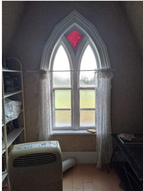
Figure 41: Interior of lancet window on east façade, not coloured and patterned glass in lancet peak
