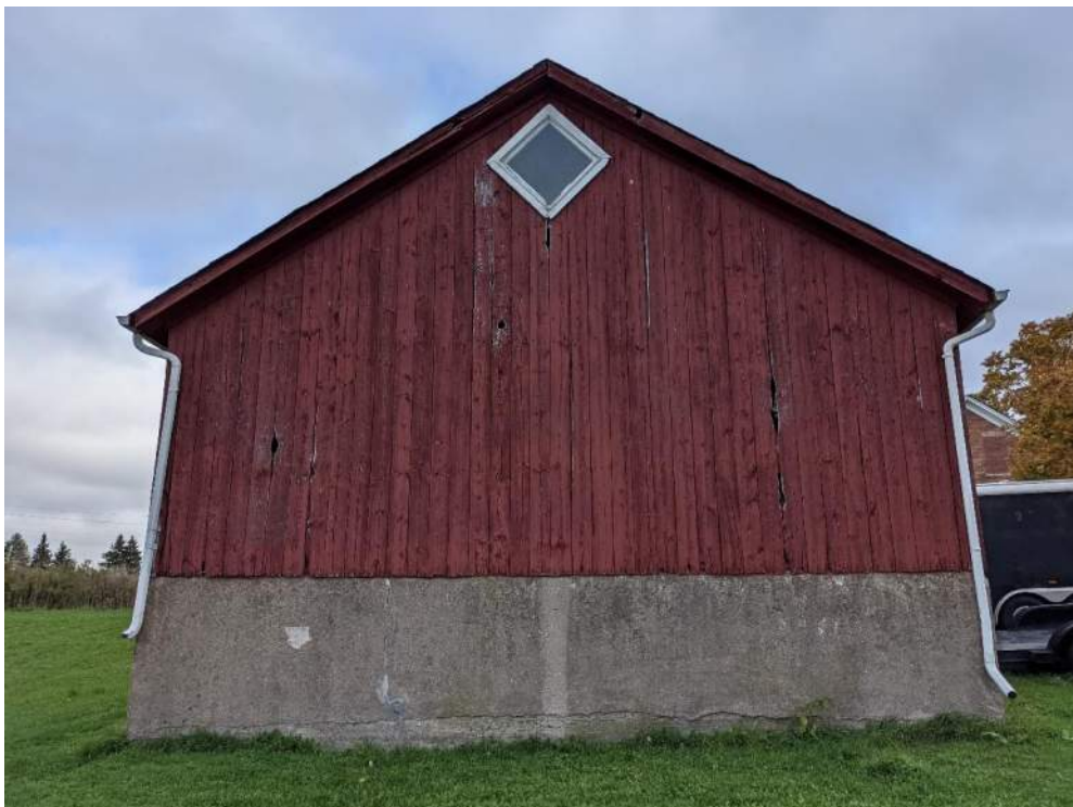
Figure 70: West elevation of the driveshed
