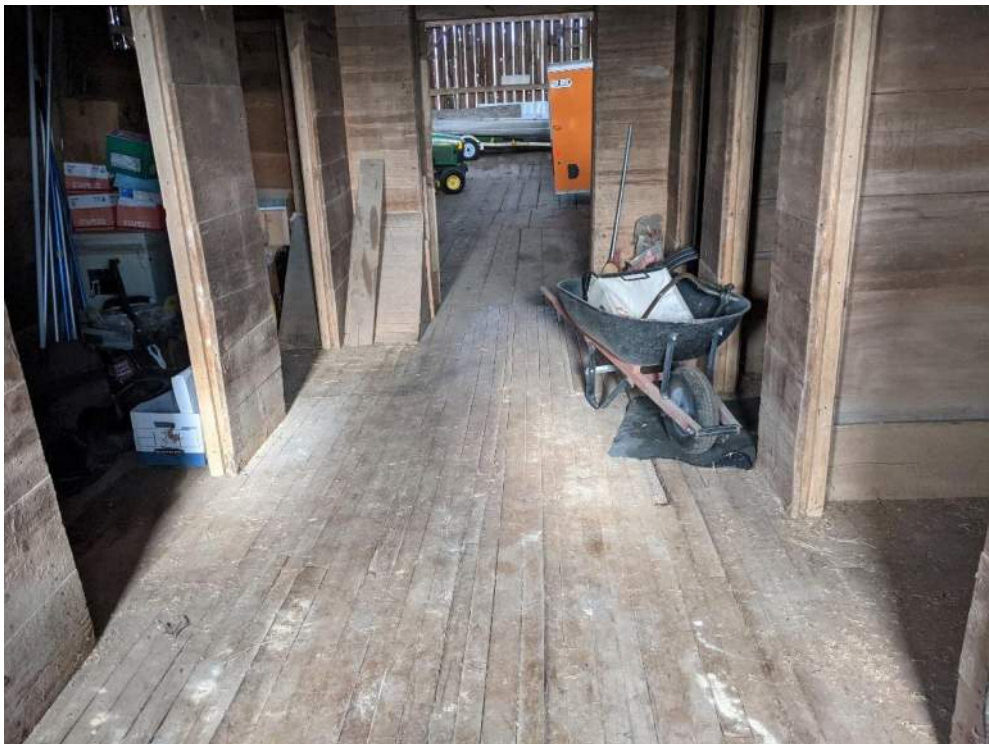
Figure 85: View inside the granary in the large barn
