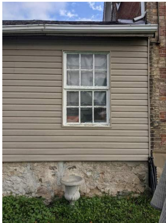
Figure 56: Six over six double hung wood sash window on the west elevation of the north addition
