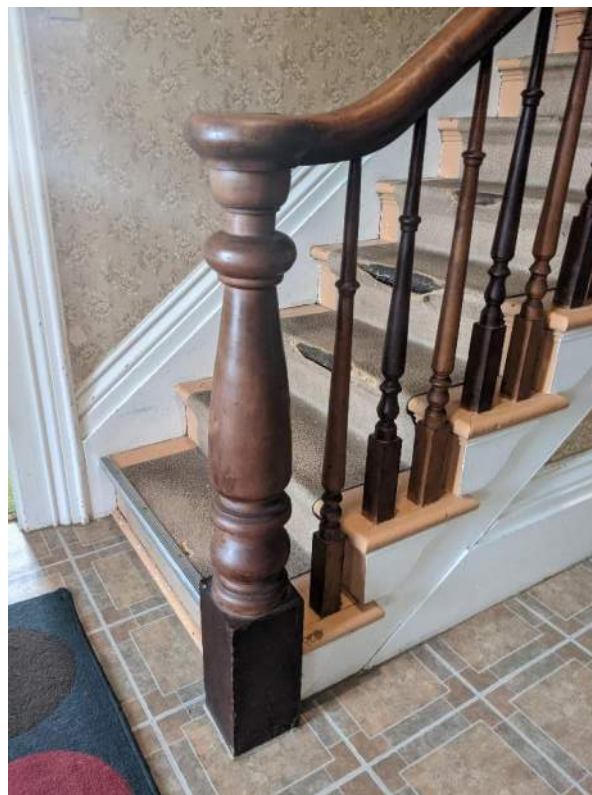
Figure 28: Staircase newel post and spindles
