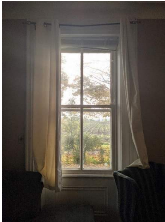
Figure 33: Wood window surround and paneling in south front room (also representative of paneling in north front room)
