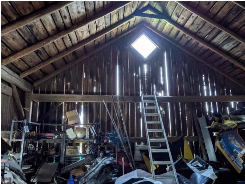
Figure 72: Dimension cut rafters
