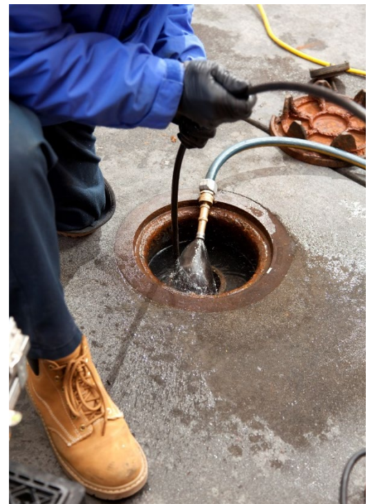
Figure 3.6-5 Example of stormwater structure maintenance (clearing/flushing).
