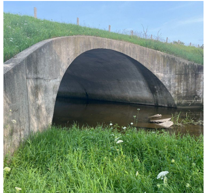
Figure 3.1-1 Example of a County CSP arch OSIM culvert (C060800, Wellington Road 6, Minto).
