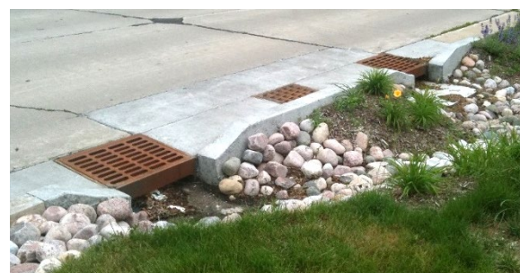
Figure 3.6-1 Example of stormwater structures (catch basins) along a curb.
