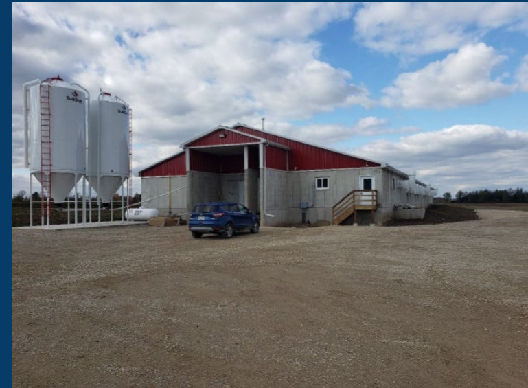
Lester Bearinger – New Hog Barn
