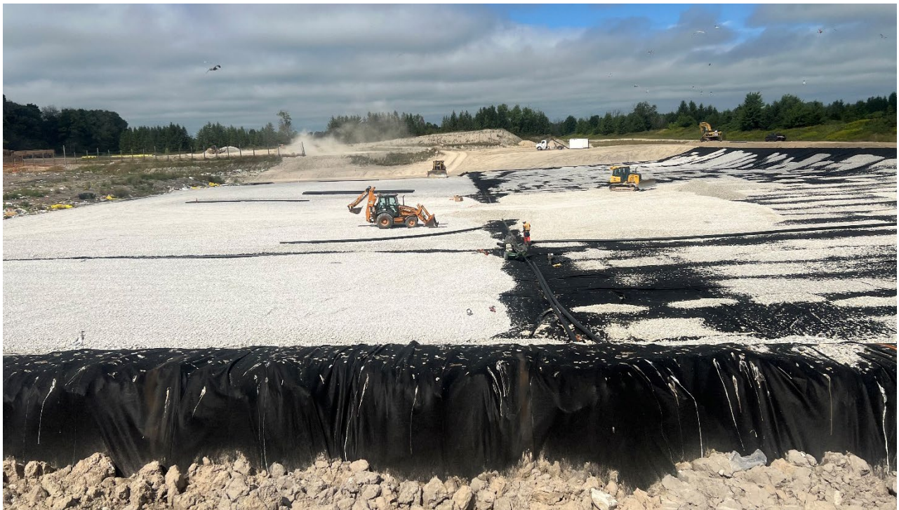
Construction of Cell 2 of Phase II at Riverstown Landfill Site
