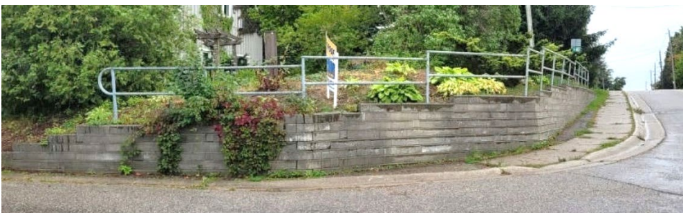
Figure 3.5-1 Example of a County retaining wall (RW036-033) along Wellington Road 36.
