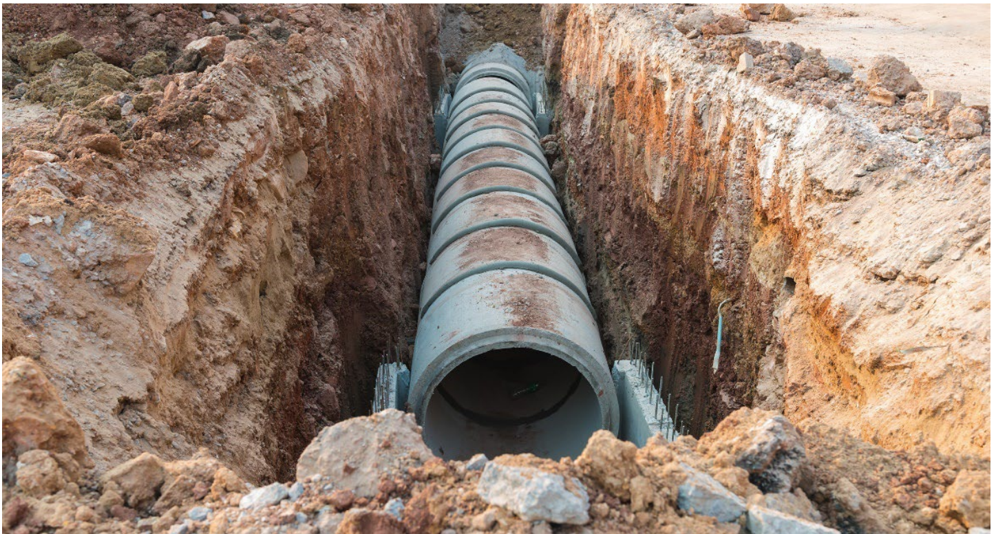
Figure 3.6-14 Example of underground stormwater infrastructure during an excavation and replacement.
