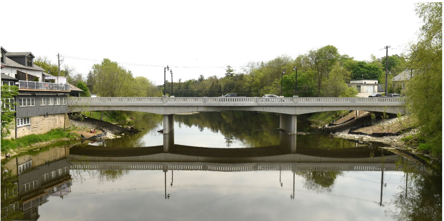
Figure 3.1-2 Example of a County concrete bridge (Badley Bridge, Wellington Road 21, Elora).
