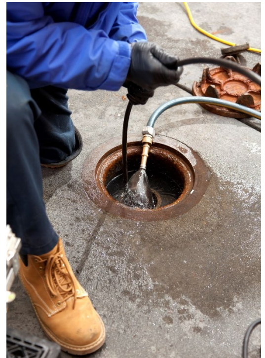
Figure 3.6-5 Example of stormwater structure maintenance (clearing/flushing).
