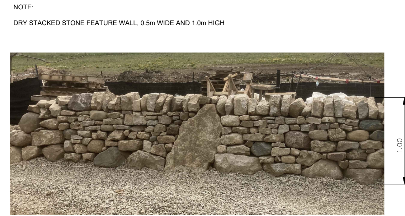
5 DRY STACKED STONE FEATURE WALL DETAIL NTS
