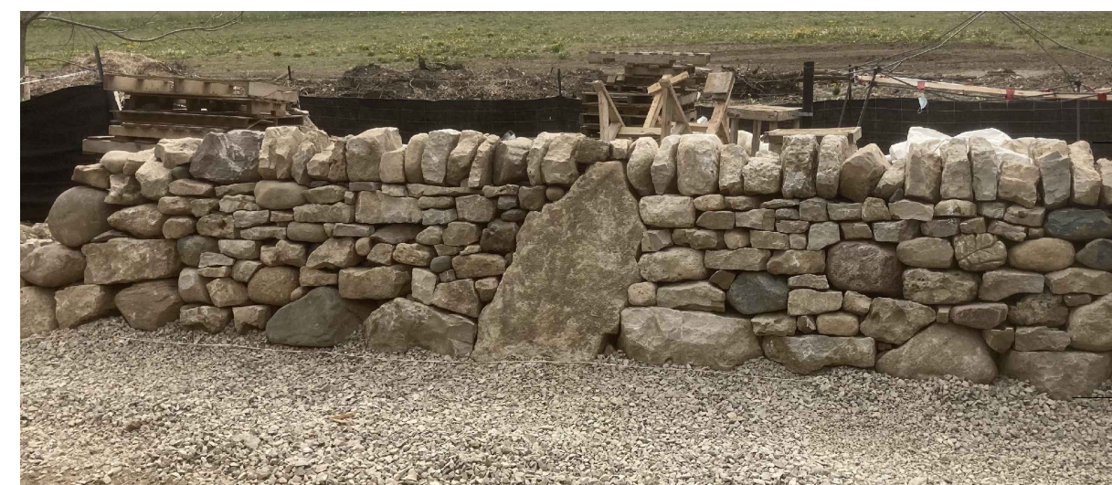
3 DRY STACKED STONE FEATURE WALL DETAIL N.T.S.
