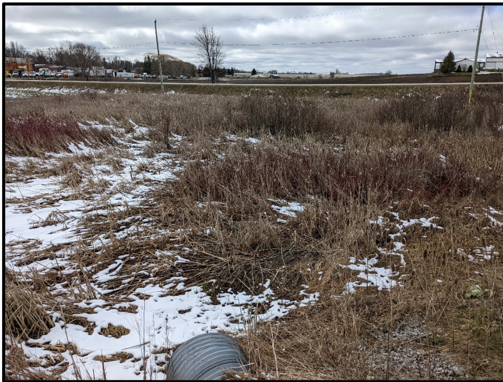
Outlet of CSP culvert to low-lying wetland area
