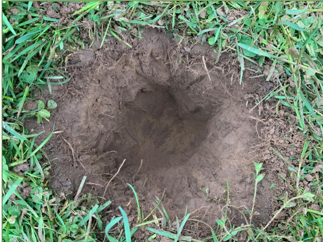
Photo 6: Typical Test Pit Facing North
