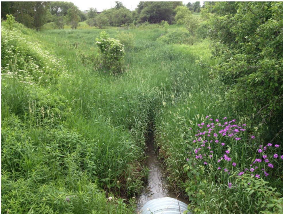
Photo No. 10: Watercourse in August, Drainage Easement Section
