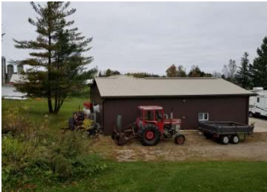
Photo 18 - View facing west of the metal clad garage located at the end of Centre Street, north of the Site.
