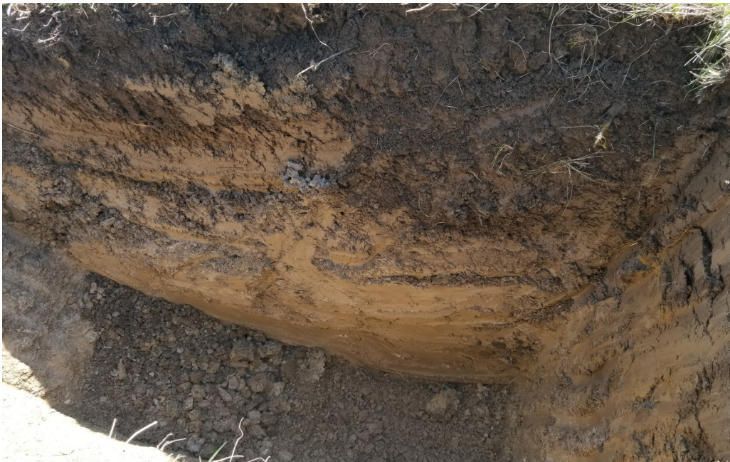
Photo 6 - TP-3 side wall.
