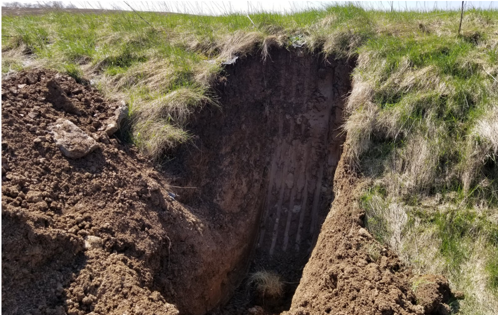
Photo 12 - TP-8 side wall.
