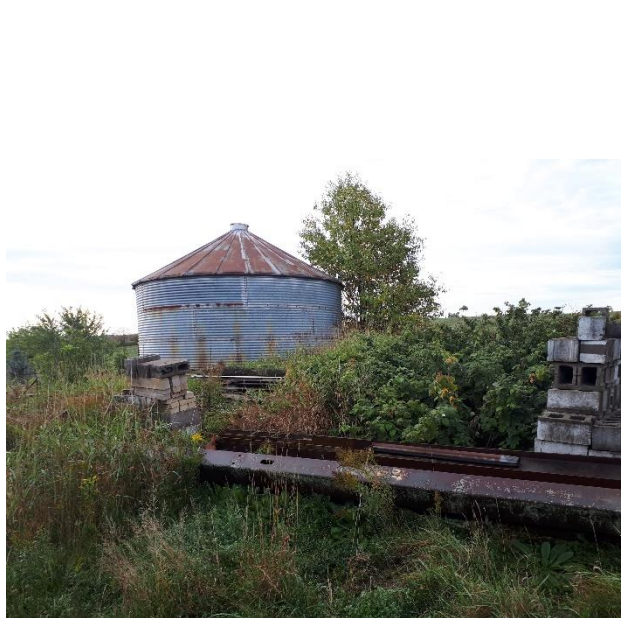
Plate 8: View of extant silo within former barn complex.
