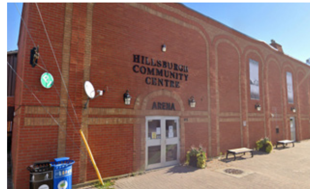
8 View of the Hillsburgh Community Centre Arena
