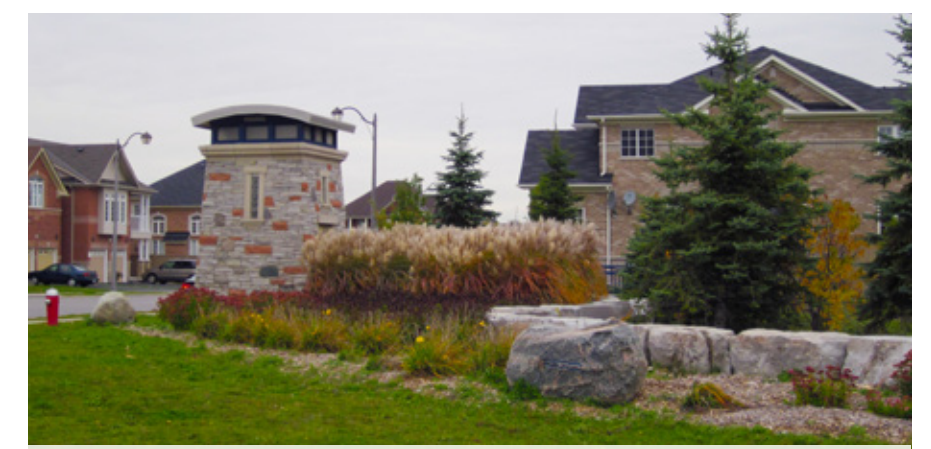
Figure 4.9: Image example of built form and landscape gateway features that emphasize the entrance into a community.
