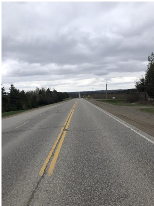
PROPOSED STREET 'A'/HOWE STREET AT TRAFALGAR ROAD NORTH – LOOKING SOUTH
