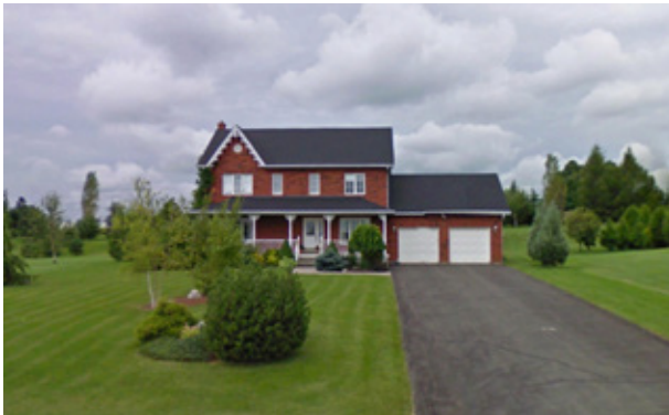
4 View of dwelling along Hill Street, showing contemporary and traditional architecture.
