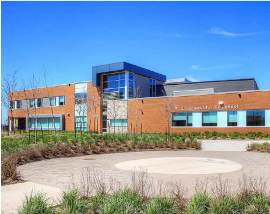
Figure 5.1: Image example of a school facade.
