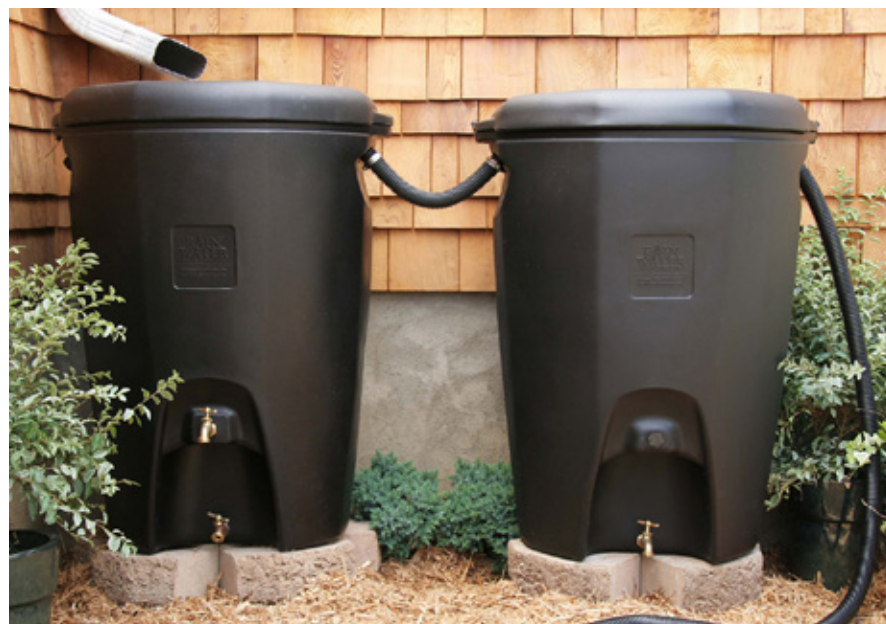
Figure 6.6: Image example of integrated rain barrels to manage rainwater runoff.
