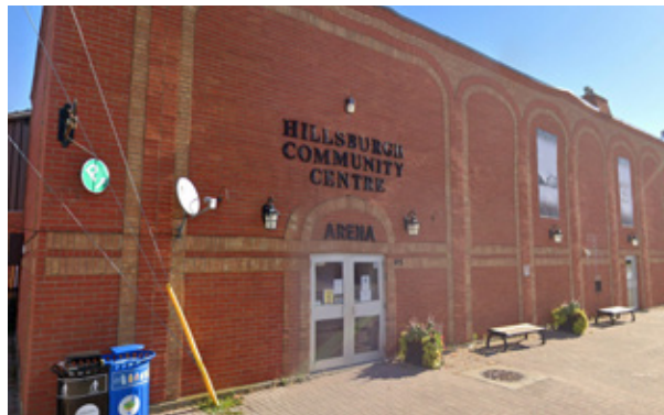
8 View of the Hillsburgh Community Centre Arena
