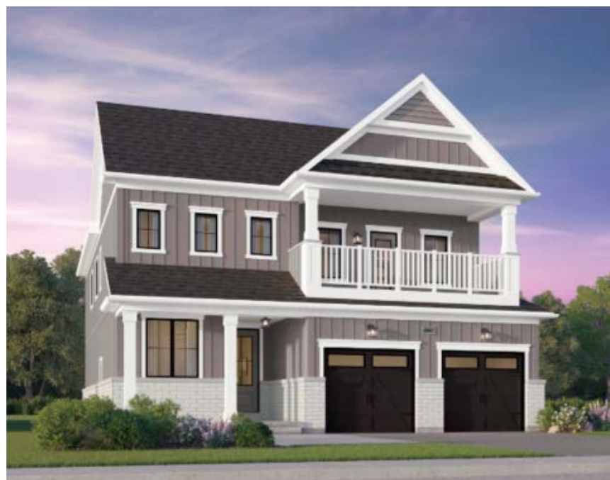
Fig.27: Single-detached home with a covered front porch, balcony, integrated garage, and architectural detailing (Source: Fergus Development Inc.)
