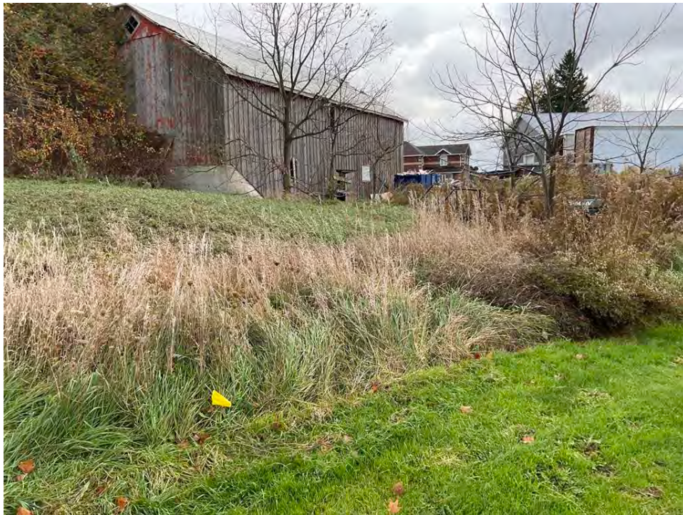
Image 9: Barn; facing southeast, October 30, 2023.
