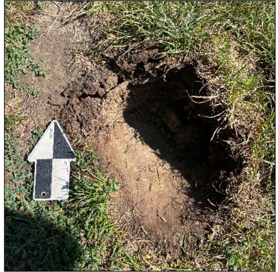
Image 22: Example of disturbed soil conditions.
