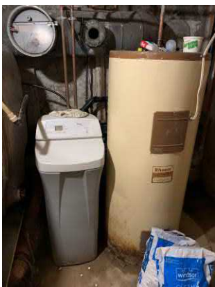
Picture 5: View of electric water heater and water softener in the clubhouse basement.
