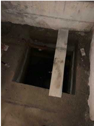
Picture 7: View of sump pit in the clubhouse basement.
