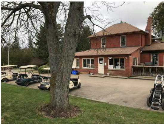
Picture 3: View of the south side of clubhouse, facing southeast
