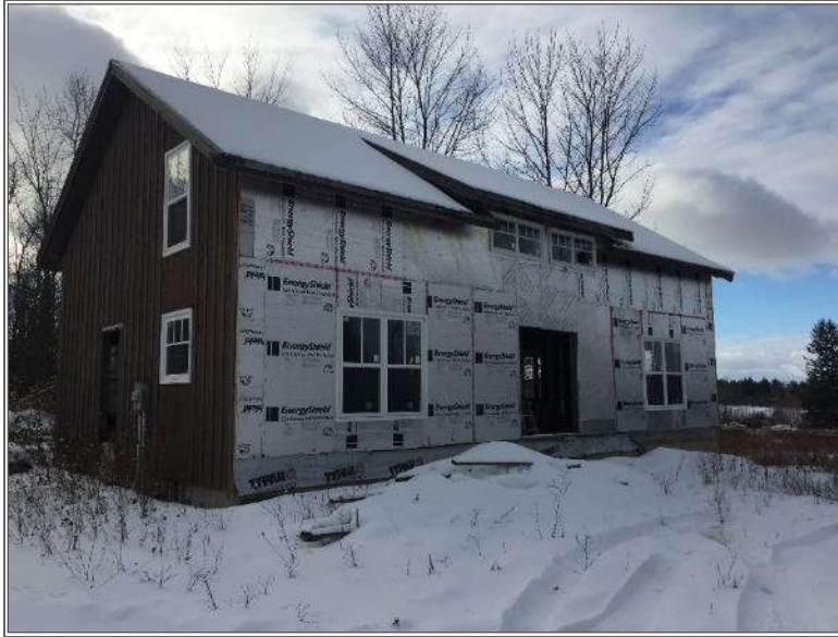
Photo 5 – Northeast elevation of Site Building C, looking southwest
