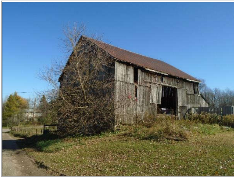
Photo 4 – Southwest elevation of Site Building B, looking northeast.
