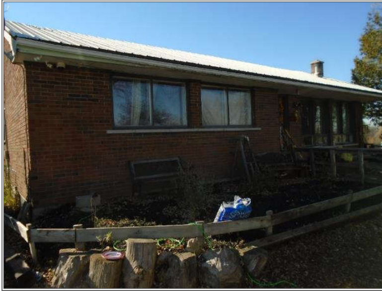
Photo 1 – Northeast elevation of Site Building A, looking southwest.
