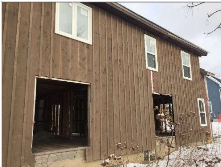
Photo 6 – Southwest elevation of Site Building C, looking northeast.
