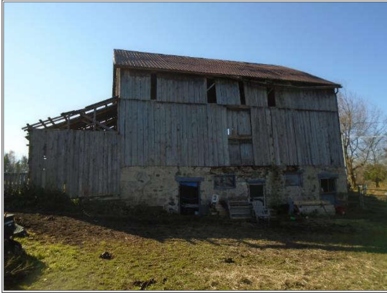
Photo 3 – Northeast elevation of Site Building B, looking southeast.
