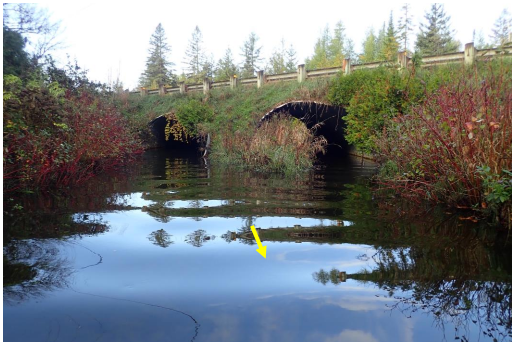
The 17 th Sideroad crossing defines the upstream extent of Reach TCR-1 .
