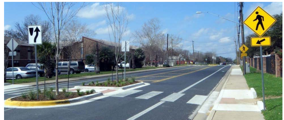
Example of a painted mid-block crossing
