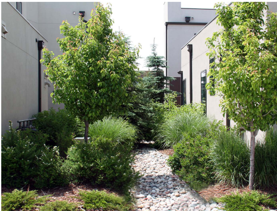
Roof downspouts help direct excess water into soakaway pits. Paired with xeriscape planting, the combination performs well in urban environments due to low-maintenance requirements.
