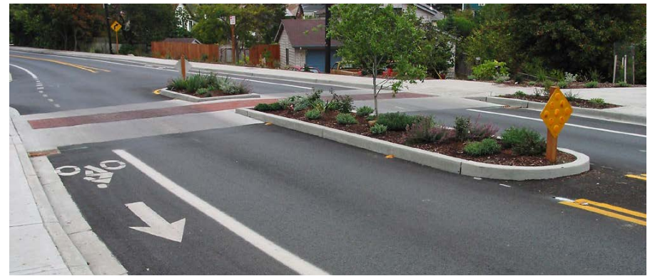
Example of a raised mid-block crossing
