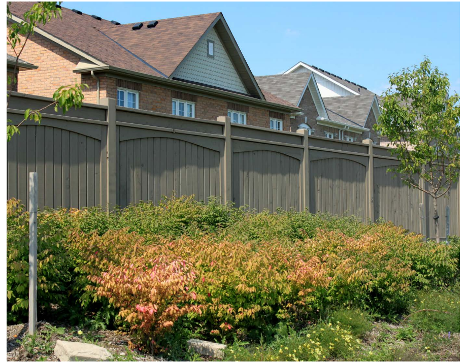
An acoustic fence protecting residential developments from traffic noise.
