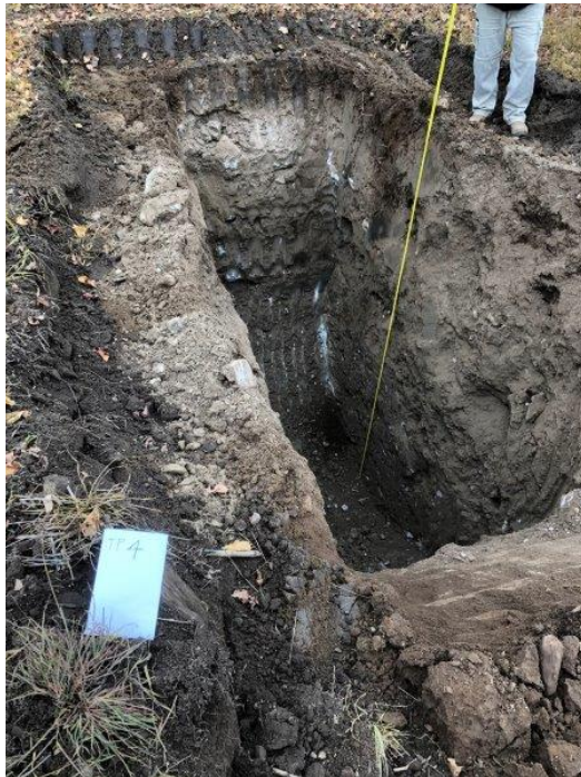
Photograph 4 – View of excavation for TP4.
