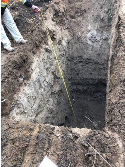
Photograph 7- View of excavation for TP7.
