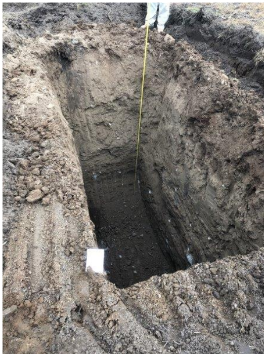
Photograph 2 – View of excavation for TP2.
