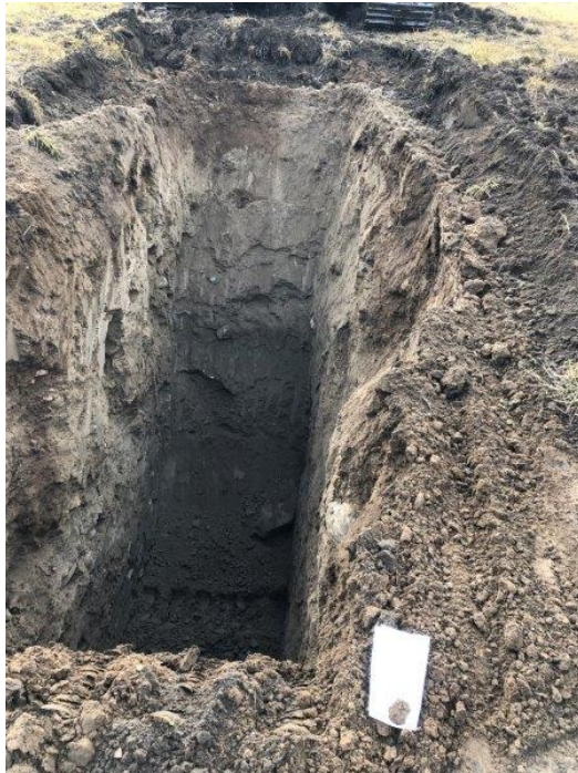
Photograph 6- View of excavation for TP6.
