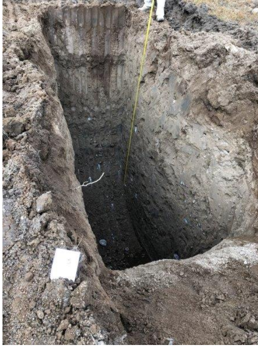
Photograph 3- View of excavation for TP3.
