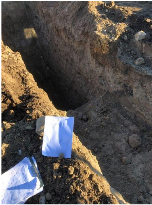
Photograph 9- View of excavation for TP9.
