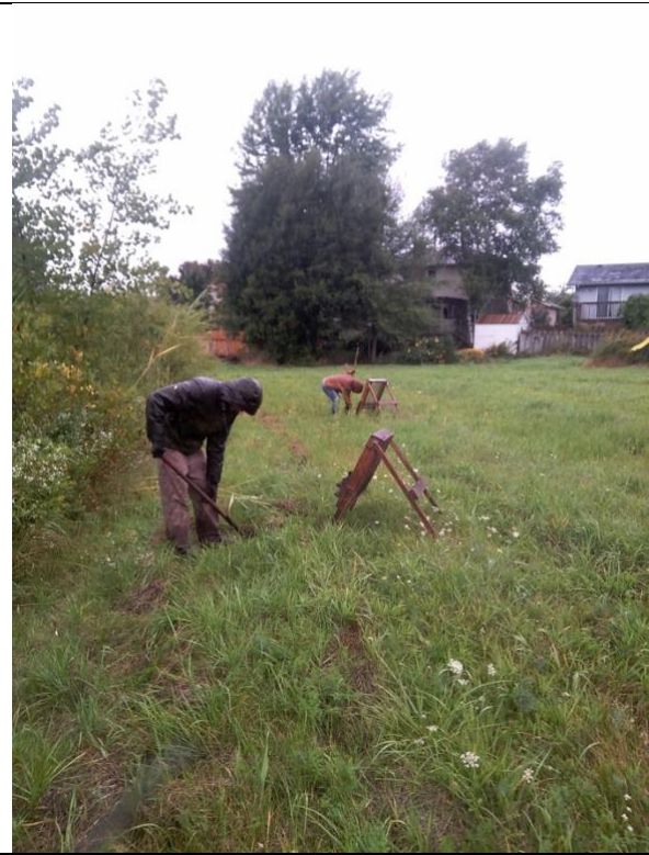
IMAGE 15 CREW AT WORK- 5M TP SURVEY
