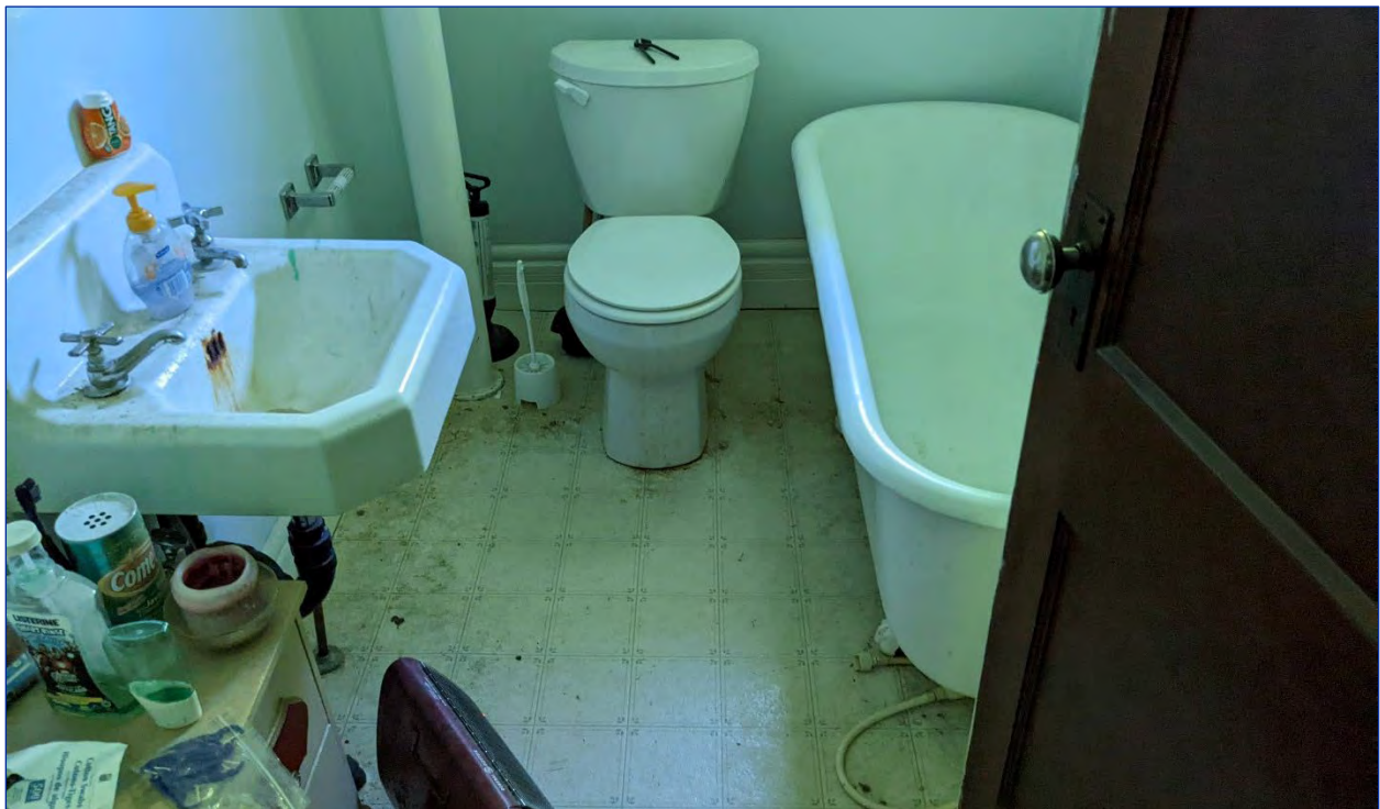
Figure 50: View of the second storey bathroom
