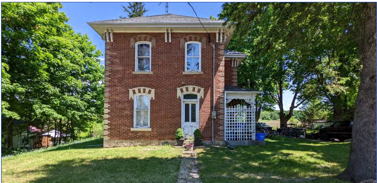
Figure 28: View of the south elevation
