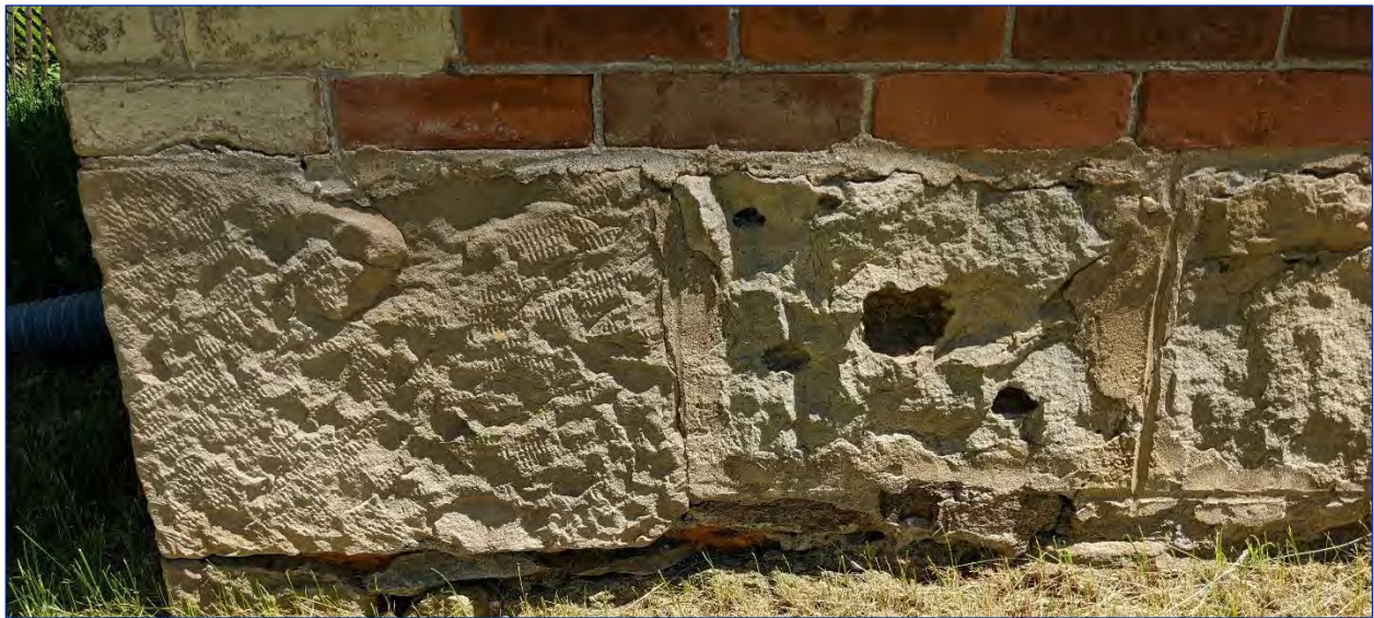
Figure 34: View of the foundation
