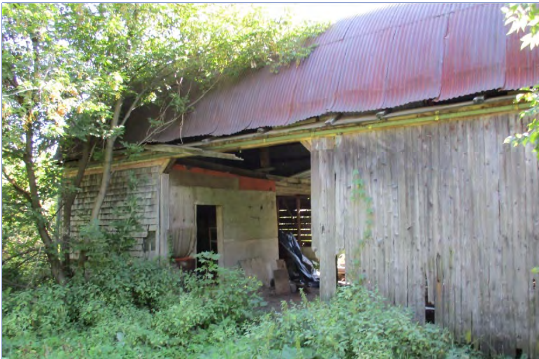
Figure 5: Image of the former drive shed 76
