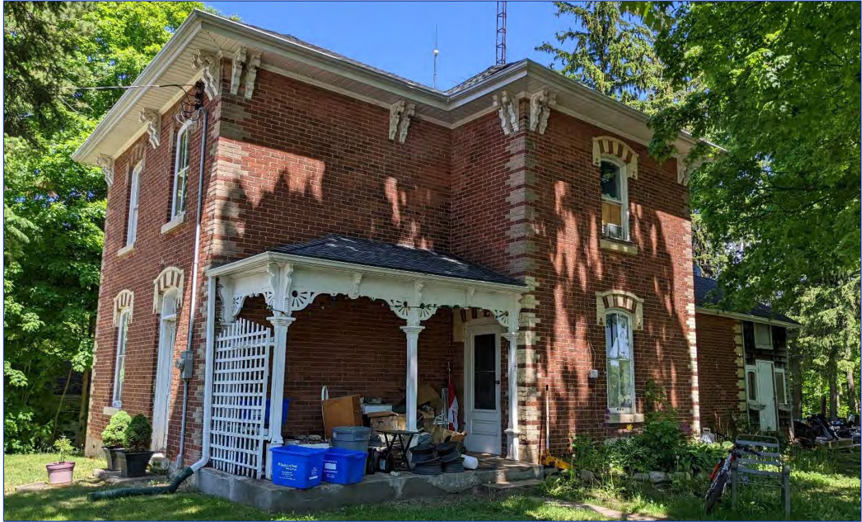
Figure 33: View of the south and east elevations
