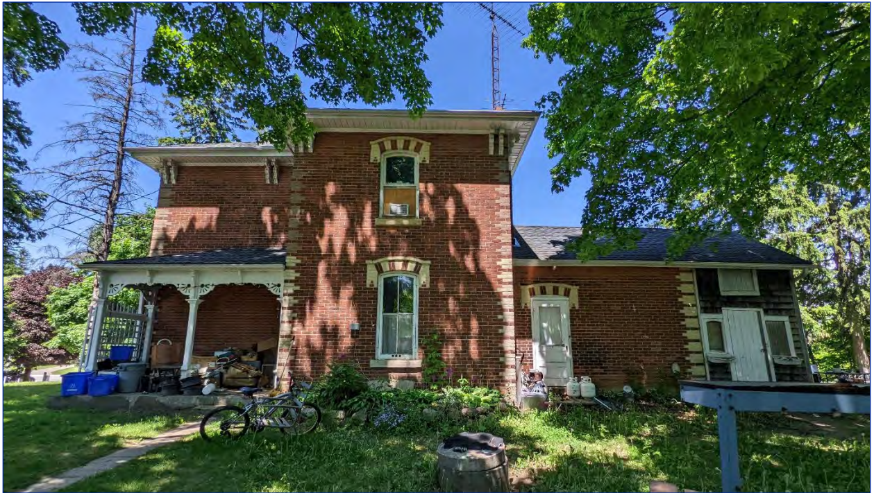
Figure 32: View of the east elevation
