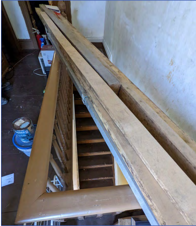
Figure 47: View of the second storey landing
