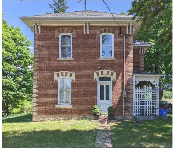
Existing heritage house to be retained.
