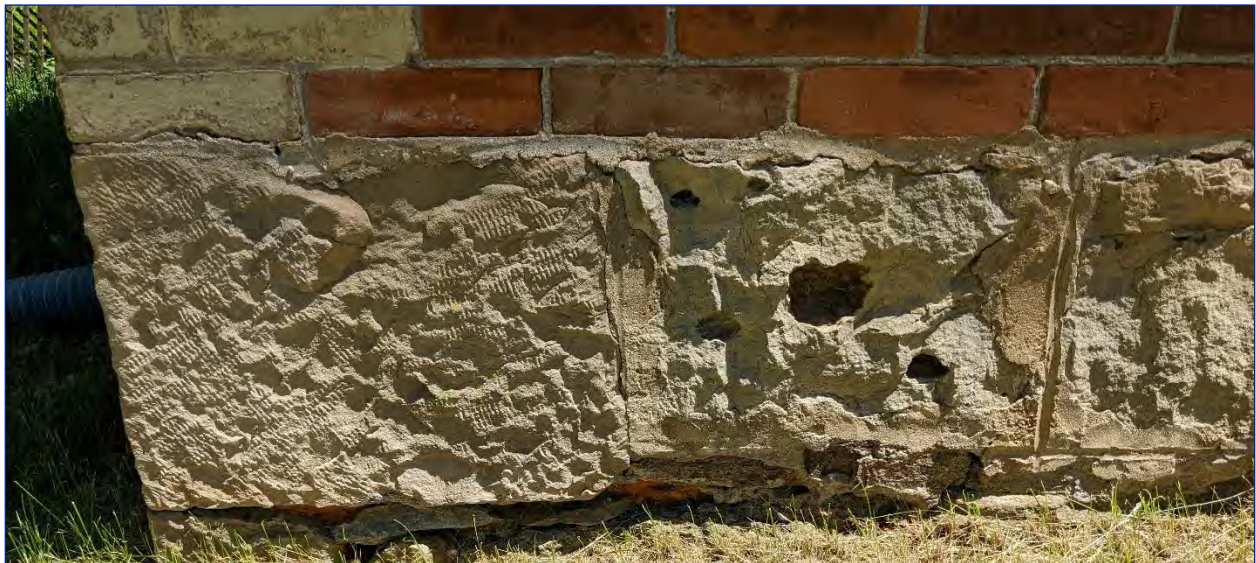
Figure 34: View of the foundation
