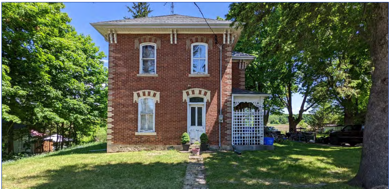
Figure 28: View of the south elevation
