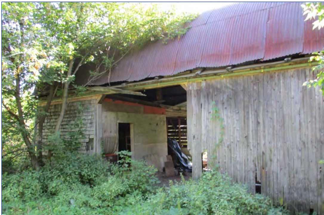
Figure 5: Image of the former drive shed 76
