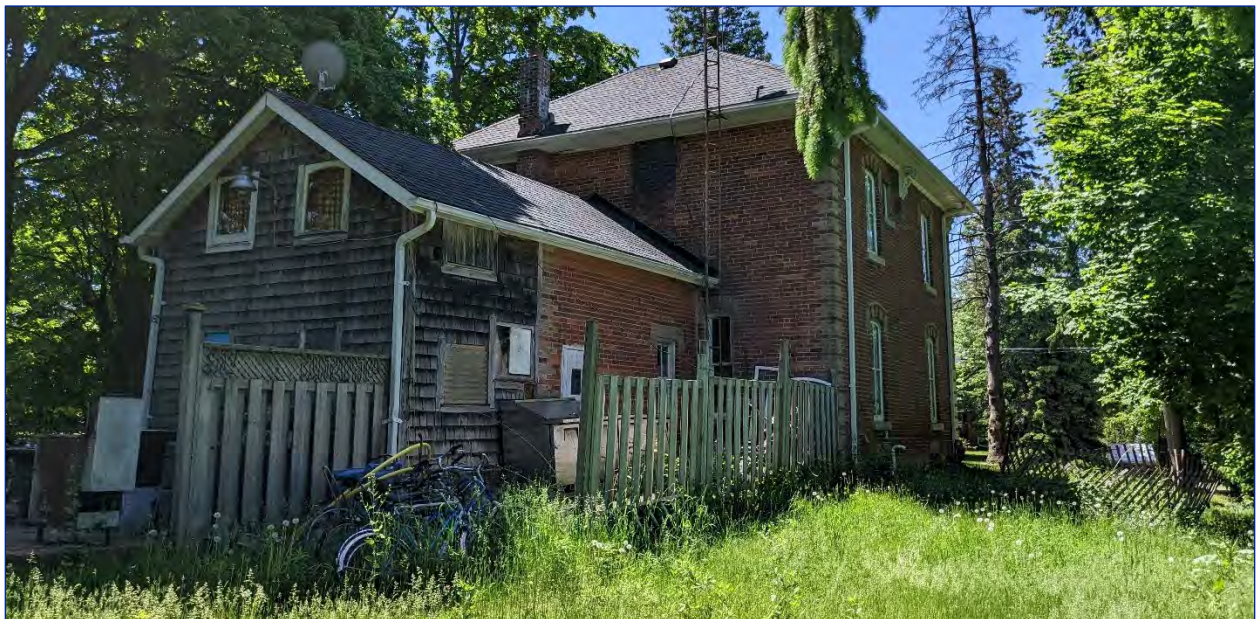
Figure 30: View of the west and north elevations
