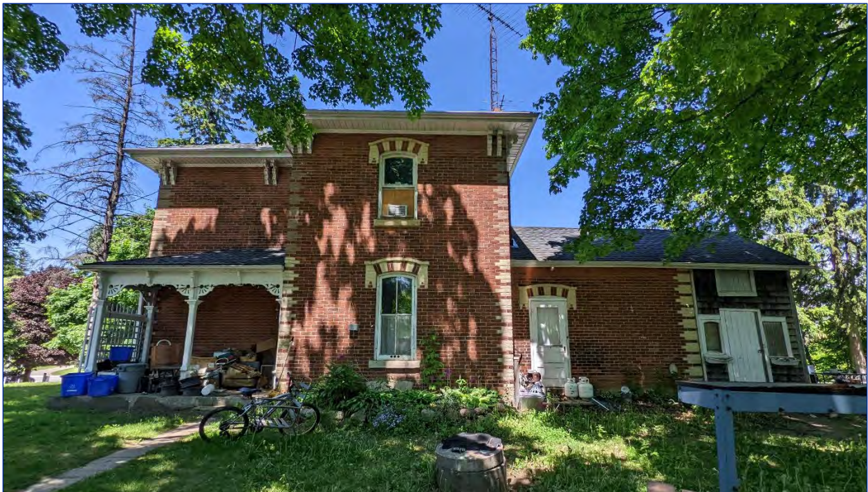
Figure 32: View of the east elevation
