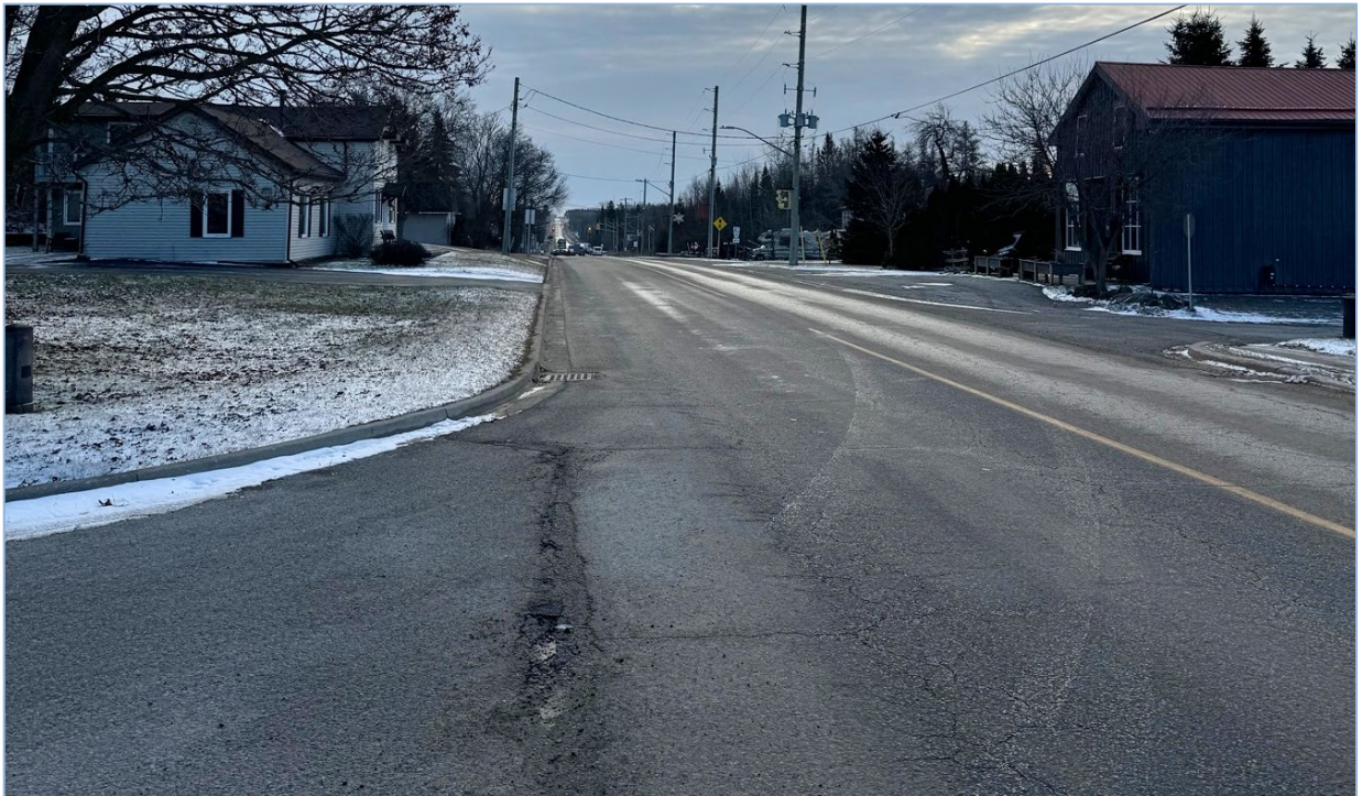
Trafalgar Road (Wellington Road 24) at Market Street – looking south
