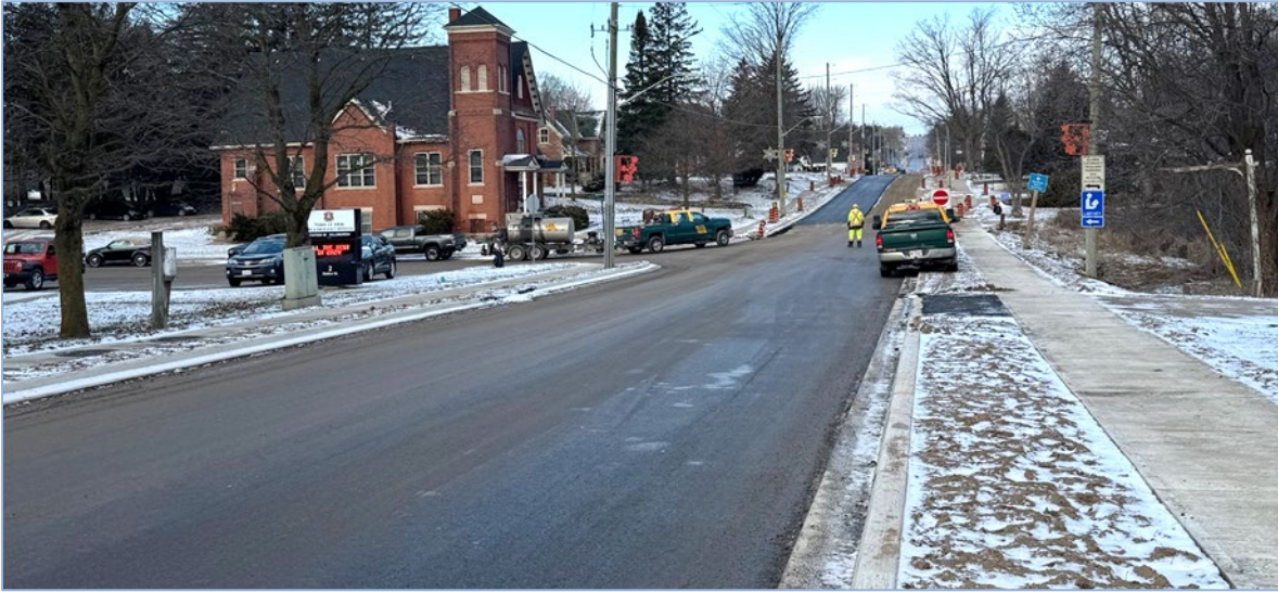
Trafalgar Road (Wellington Road 24) at Station Street – looking north
