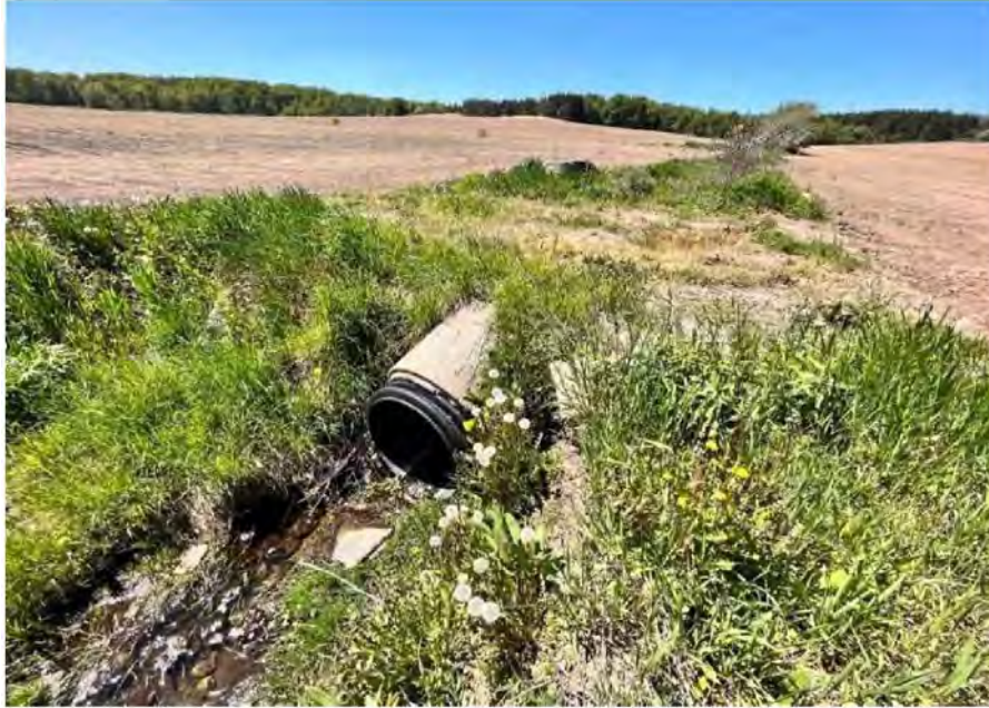
Image 1 – Large Access Culvert Along North-South Watercourse.
