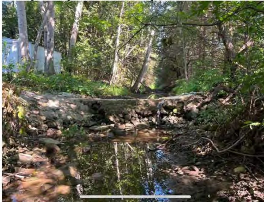
Image 2 - Small concrete dam structure Along North-South Watercourse.
