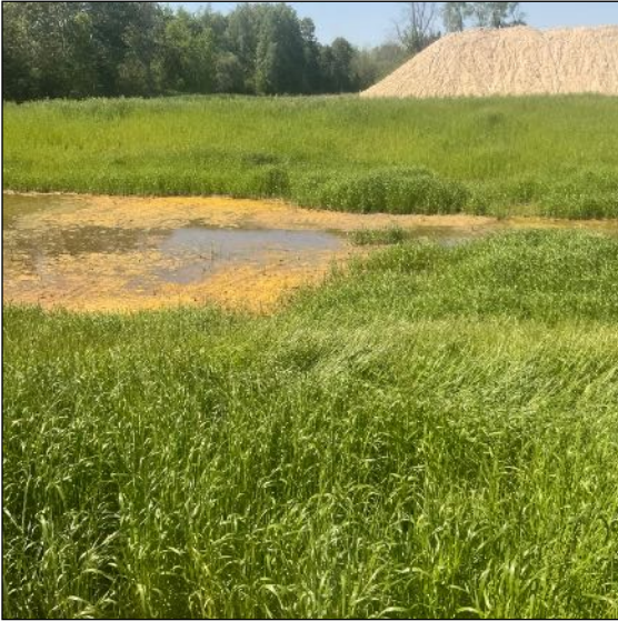
Image 5: Excavated and graded drainage channel.
