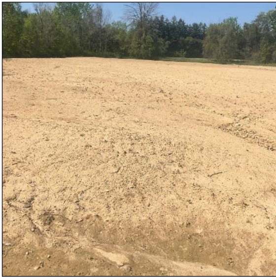
Image 7: Area of disturbance related to channel excavation, area subject to combination survey of 5 m Pedestrian Survey and 5 m Judgmental Test Pit Survey.
