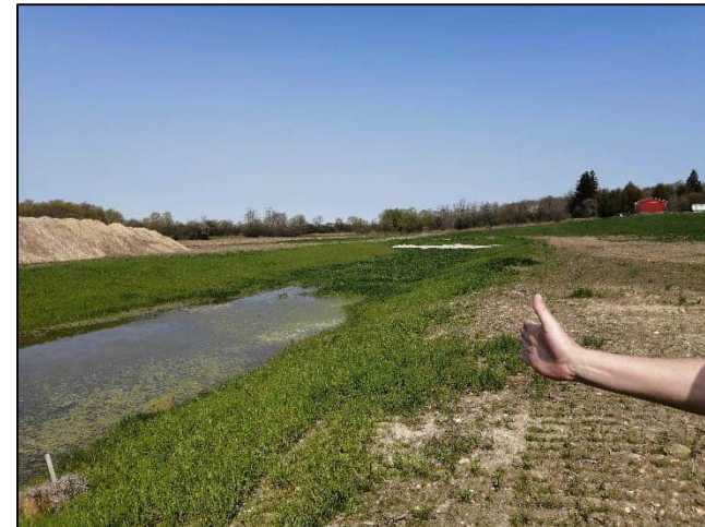
Photo 6. Standing water within Kurtz Drainage Works (Branch C at area of proposed crossing) (10 May 2023).
