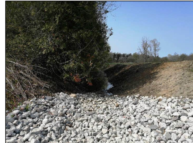
Photo 8. Ditch B (former Kurtz Drainage Works Branch F) (10 May 2023).
