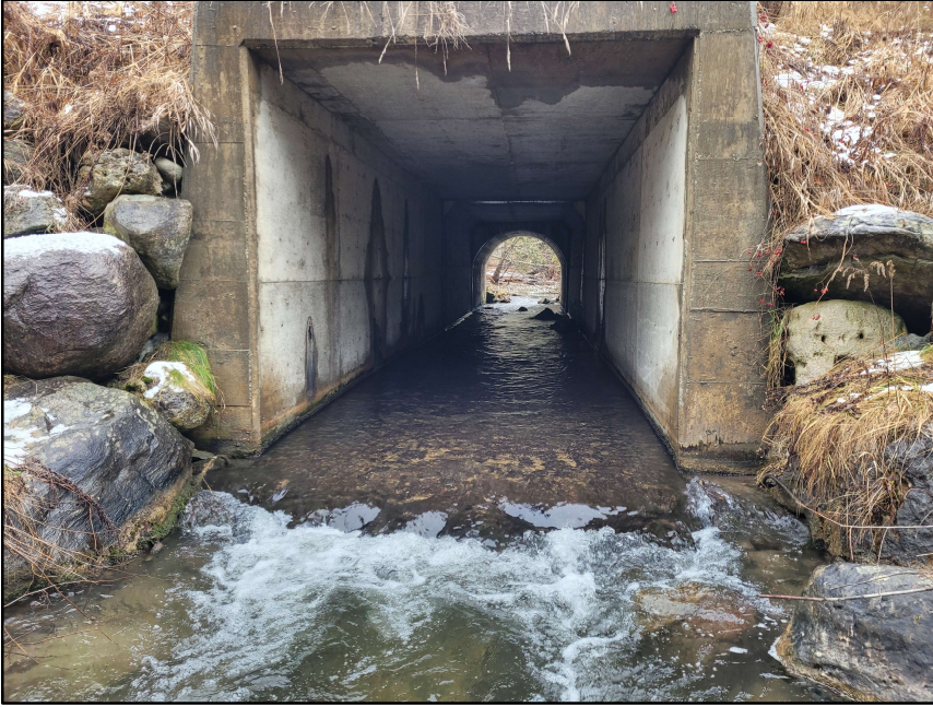
Photo 1. Facing WNW, downstream of Wellington 22. Elevation change creating a minor drop into a plunge pool at downstream extent of culvert.
