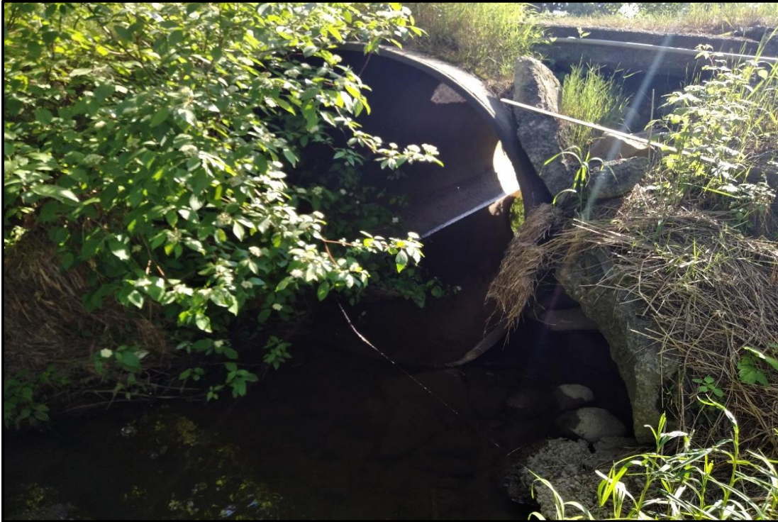
Photograph 1. Downstream View of the Culvert Under the Gibson Property Driveway (June 12, 2025)
