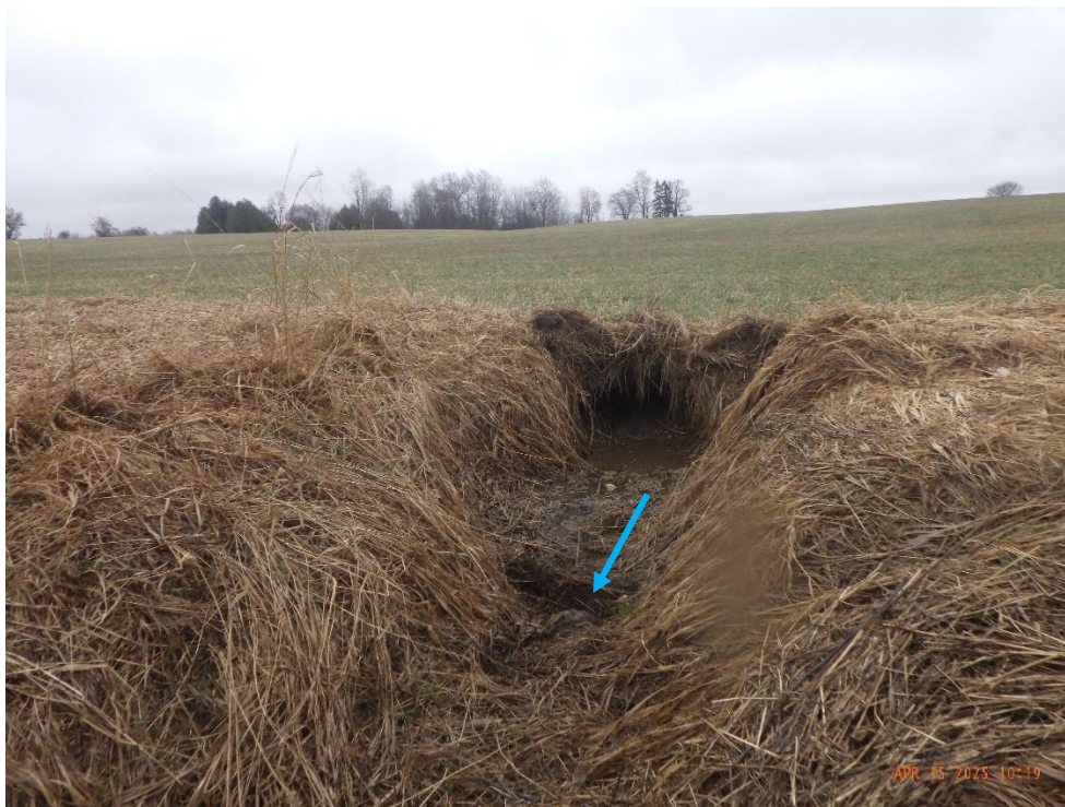
Photograph facing above the right bank highlighting a tile drain from adjacent agriculture field. The tile drain diameter was 0.14m.
