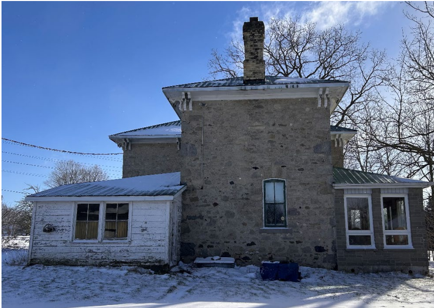
Figure 9 – rear façade (north elevation)
