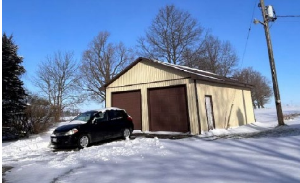
PHOTO 7: Metal Clad Frame Garage (MHBC 2025)
