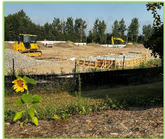
Elora Waste Facility under construction
