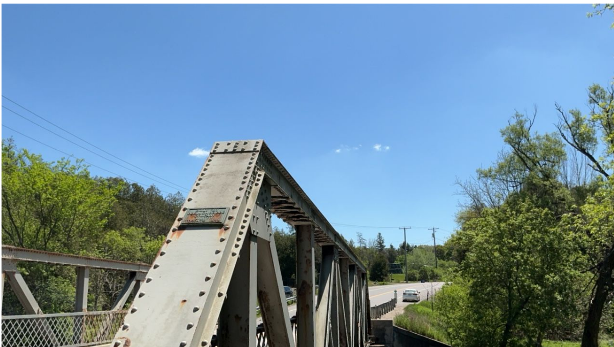
West top chord.
