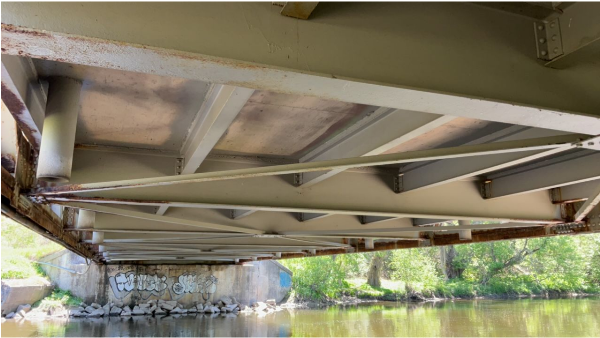
North floor beams.
