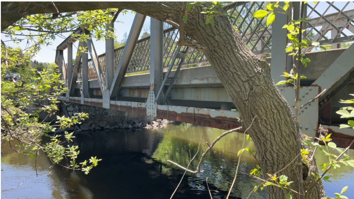
East exterior soffit.
