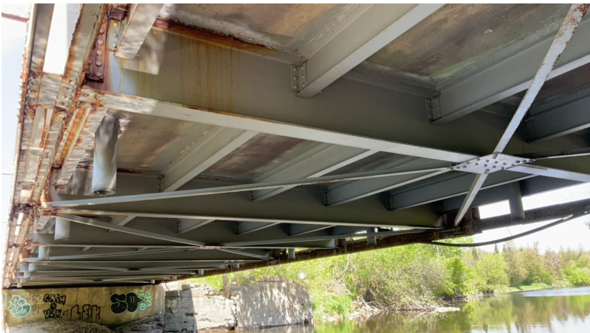
South floor beams.
