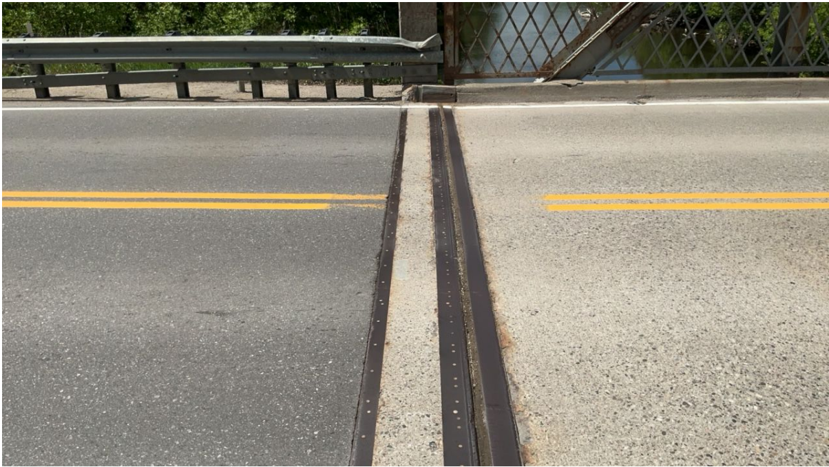
South end dam.
