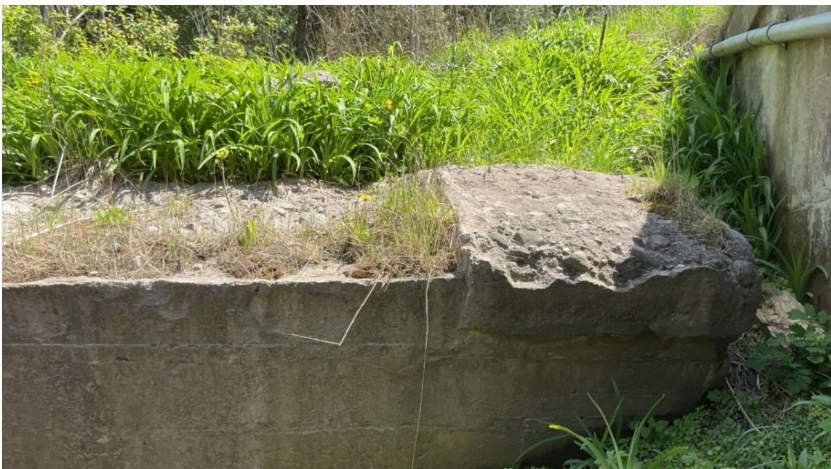
SE embankment with previous bridge structure.
