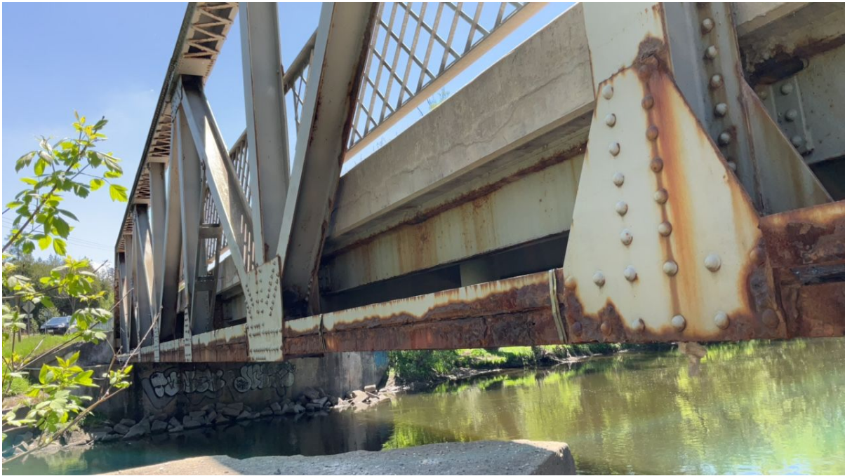
East bottom chord.
