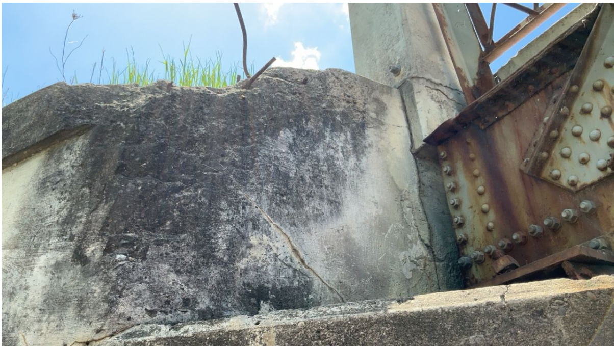
SW cracking.
