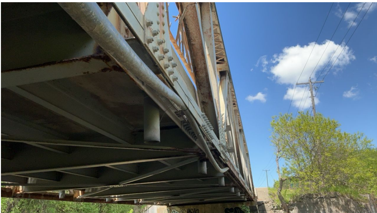
Utilities along East chord.
