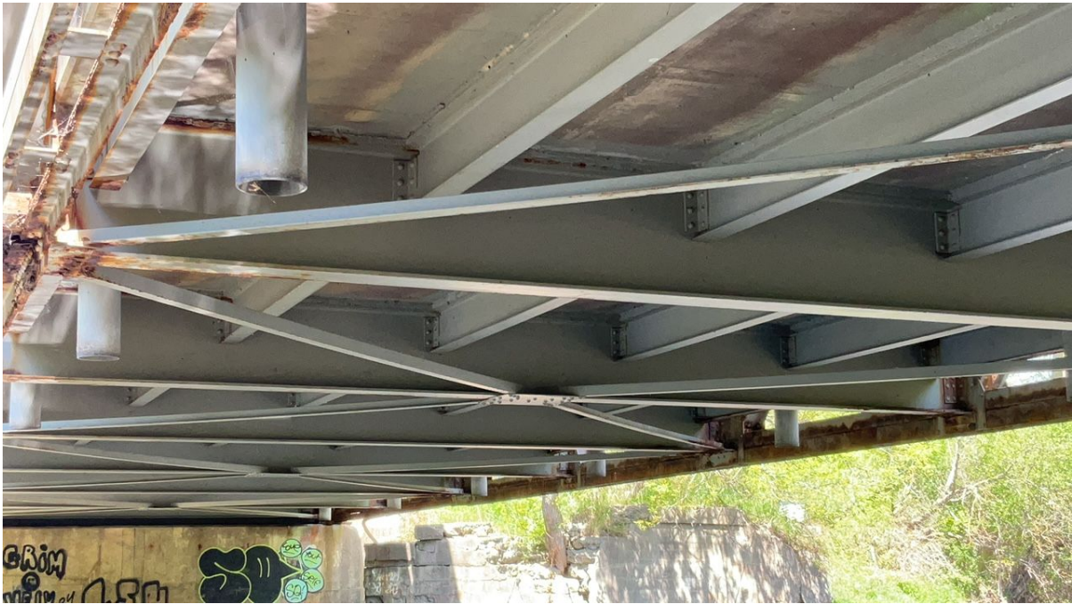
South bracing middle.
