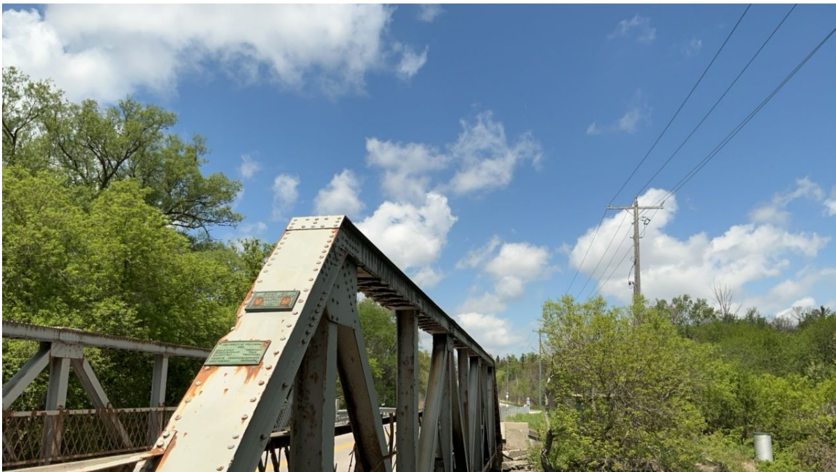
East top chord.
