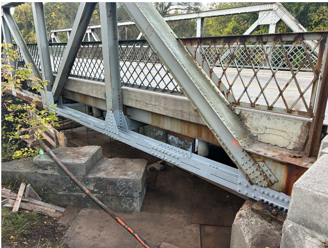
NE bottom chord repair
