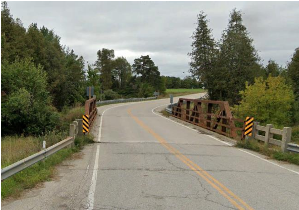
Figure 30: Flax Bridge (Google Streetview).
