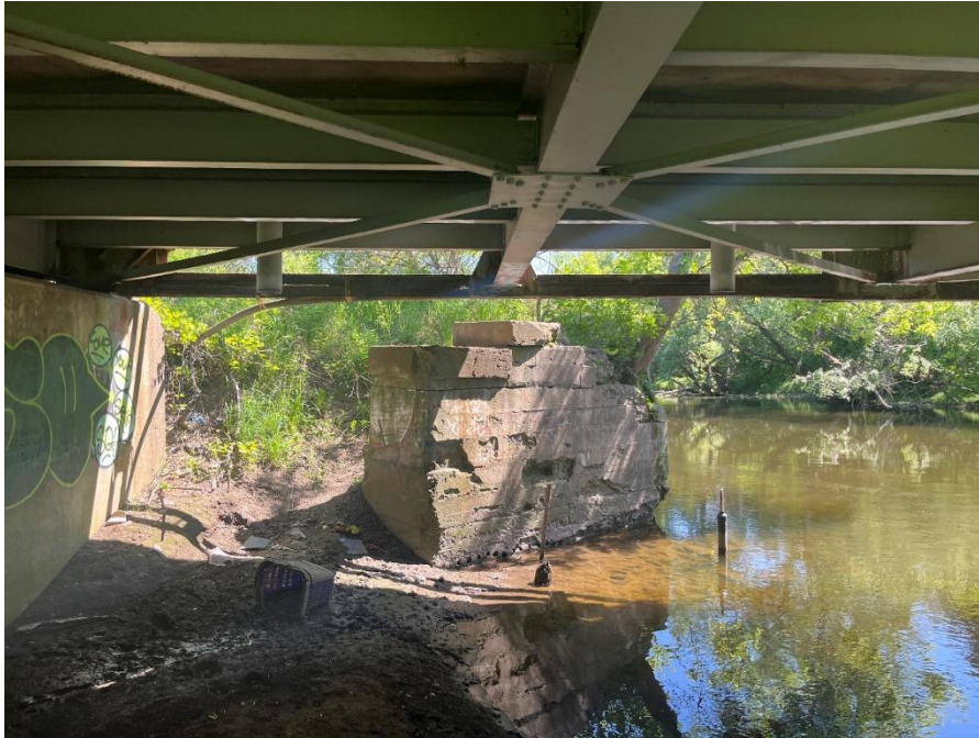
Figure 13: Under the subject bridge looking east at remnants of the previous bridge (A.S.I., 2024).
