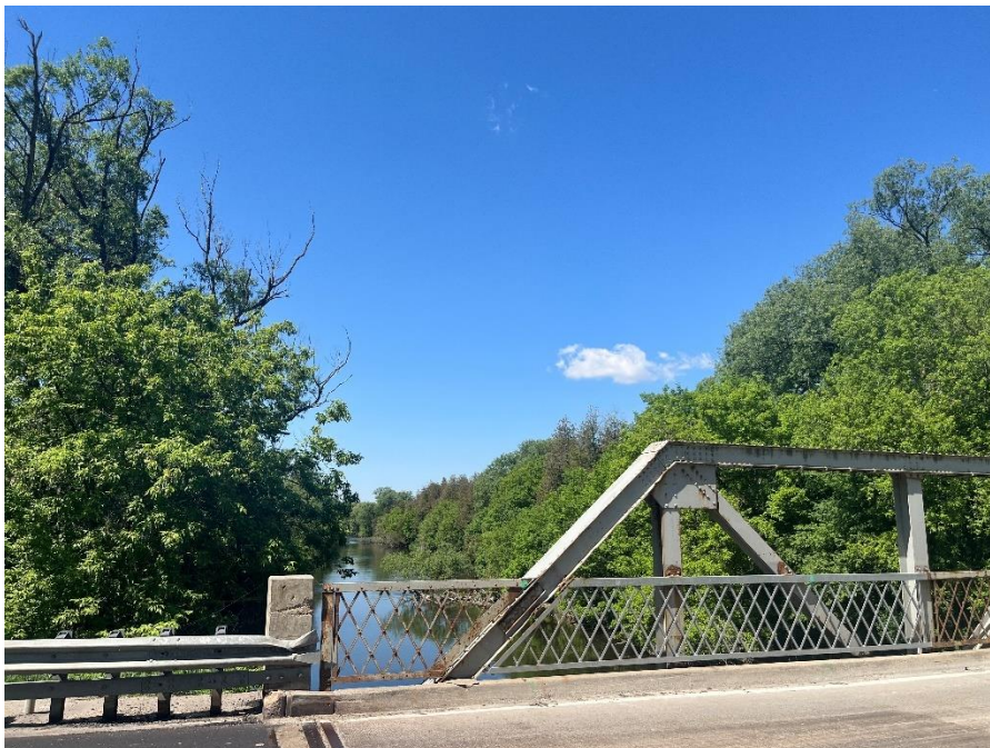
Figure 12: Detail of the steel lattice railing (A.S.I., 2024).
