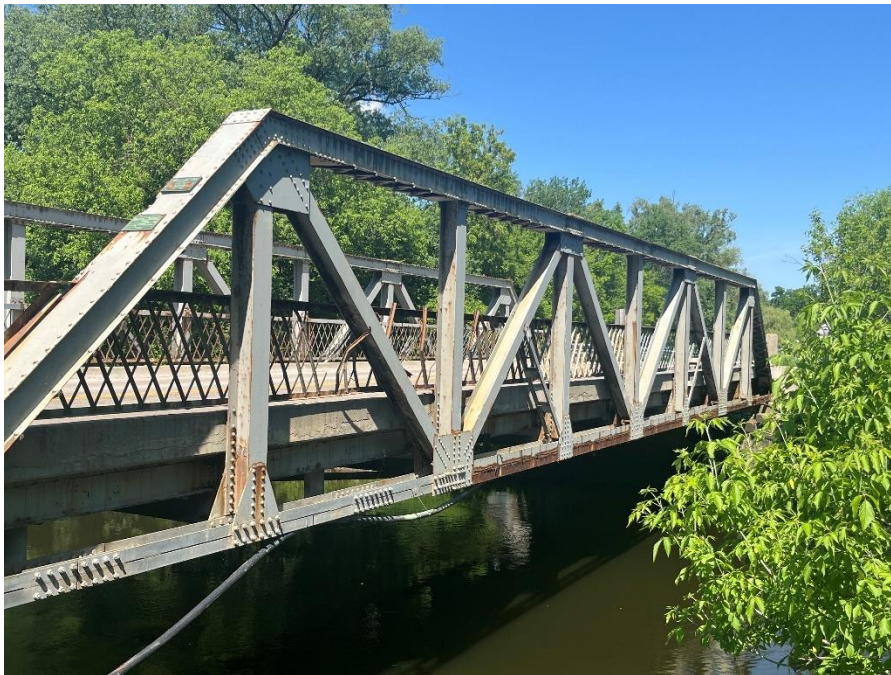
Figure 10: Oblique view of the east elevation, looking south (A.S.I., 2024).
