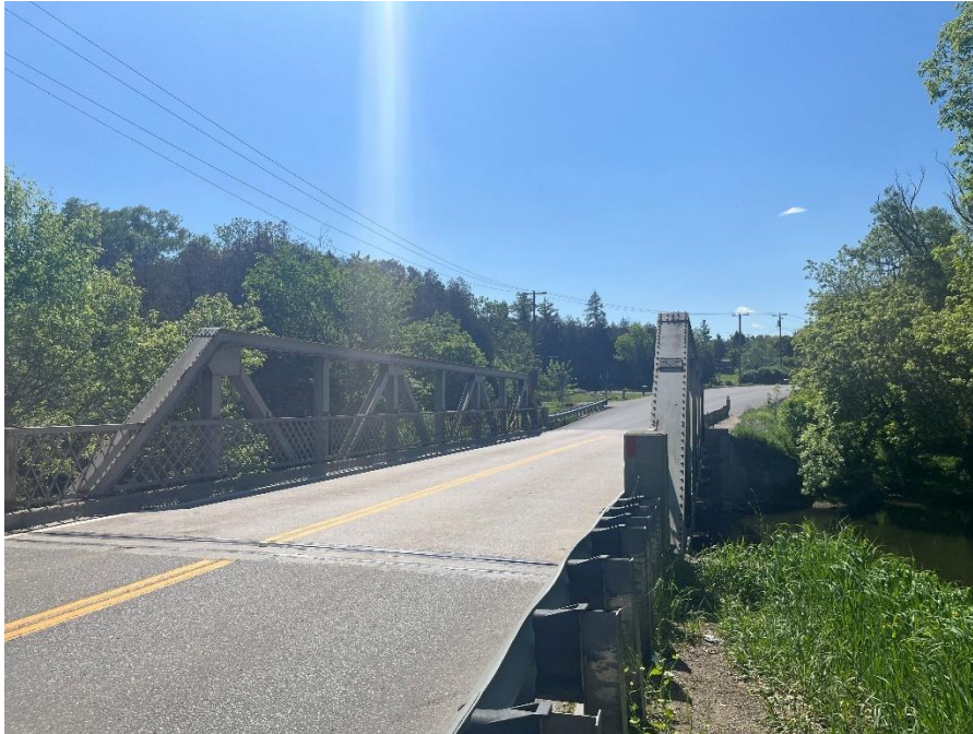
Figure 17: View of the bridge deck from the northern approach (A.S.I., 2024).
