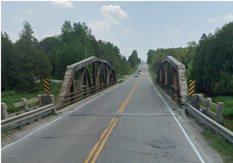
Figure 26: Bosworth Bridge prior to replacement (Google Streetview).
