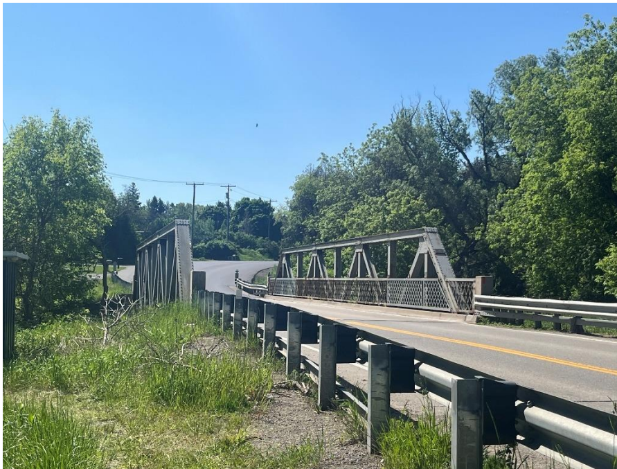
Figure 19: South facing approach to the subject bridge surrounded by vegetation (A.S.I., 2024).
