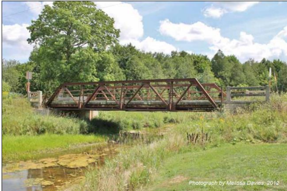
Figure 25: Mallet River Bridge (Melissa Davies, 2012).
