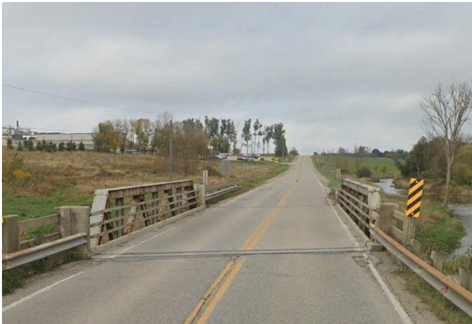
Figure 28: Rothsay Bridge (Google Streetview).
