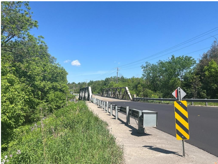
Figure 18: View of southern approach to bridge, looking north (A.S.I., 2024).
