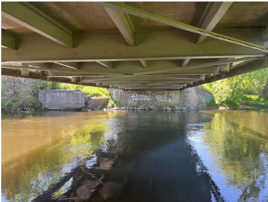
Figure 14: View to the southern abutment, looking south (A.S.I., 2024).
