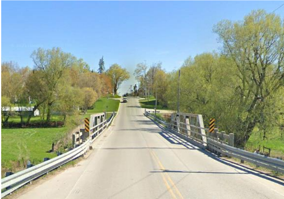
Figure 29: Moorefield Bridge (Google Streetview).
