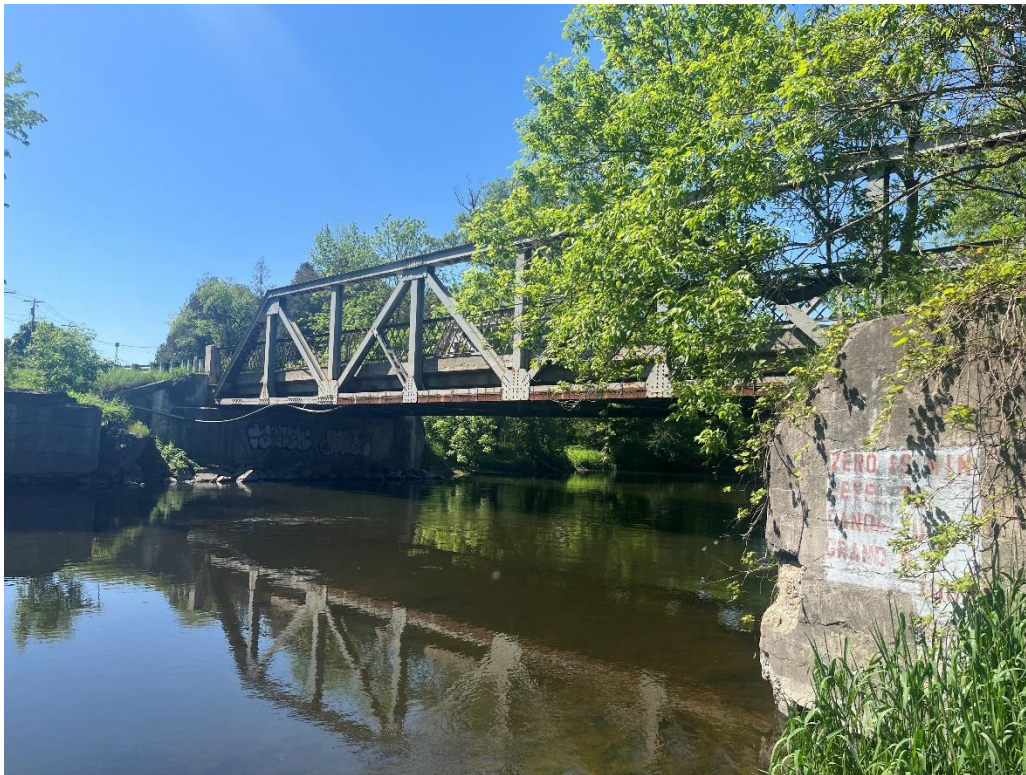
Figure 1: Blatchford Bridge, looking west (A.S.I. 2024).
