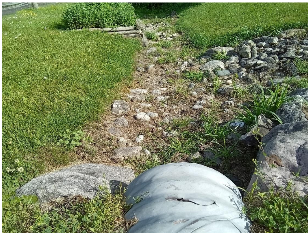
Image 4: Study Area – disturbed: culvert.
