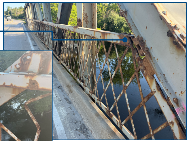
East Traffic Barrier
