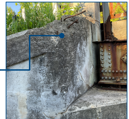
South Ballast Wall
