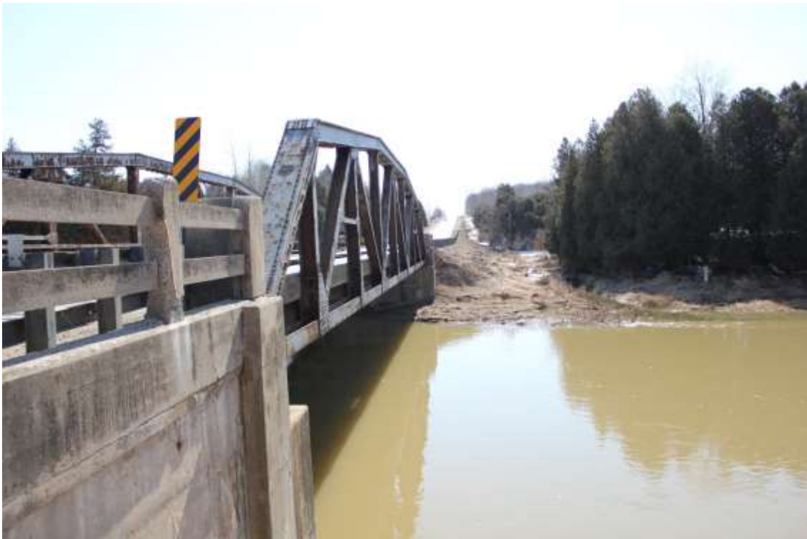
Photo 6: Downstream face looking east
