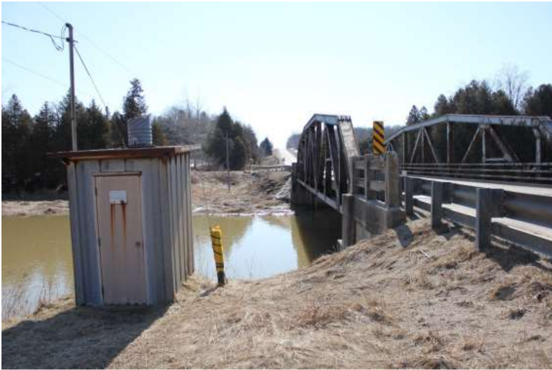
Photo 3: Upstream face looking east
