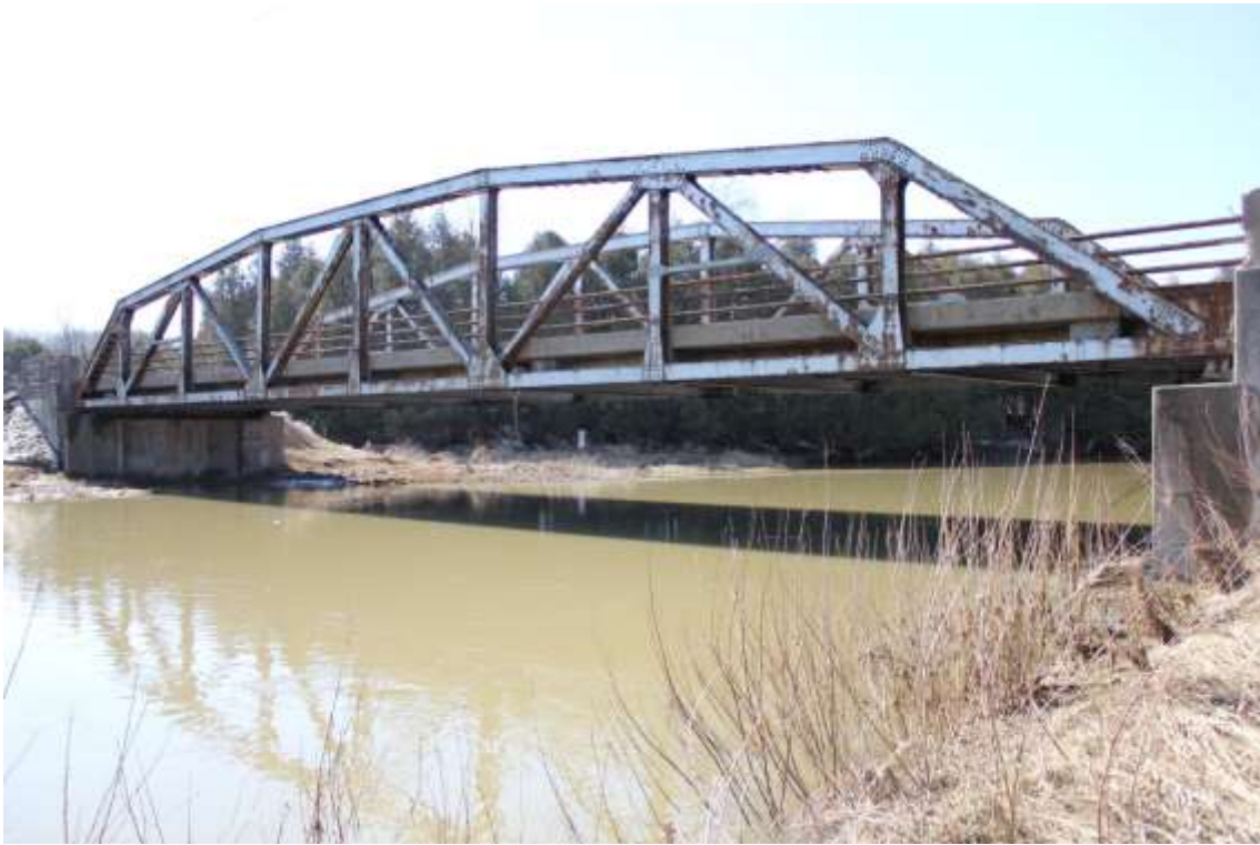
Photo 1: Upstream (north) face of the structure
