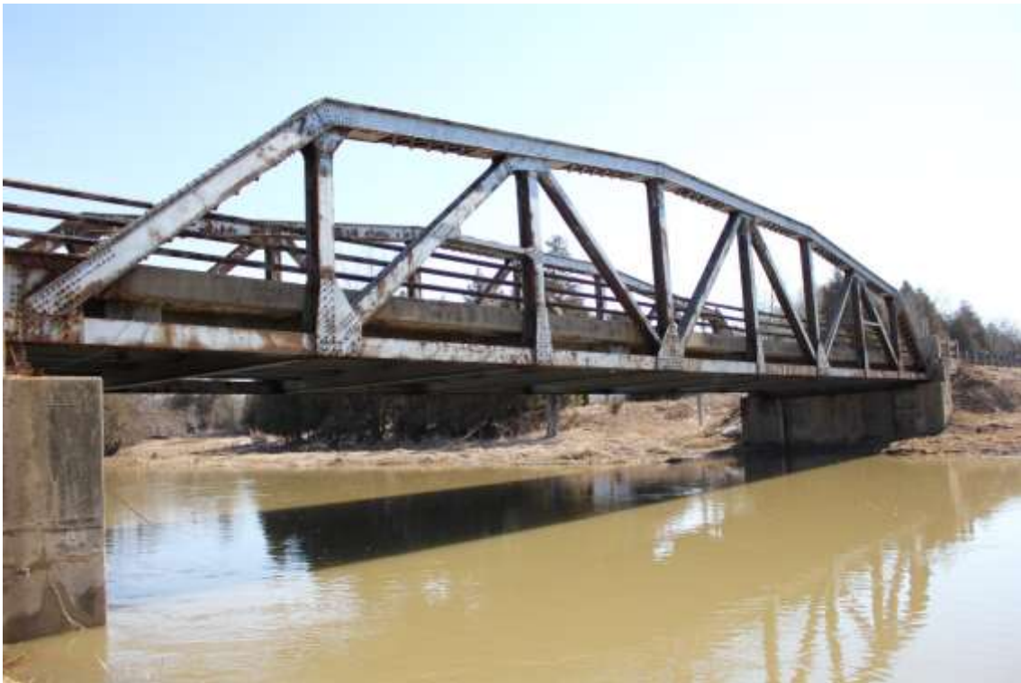
Photo 4: Downstream (south) face of the structure
