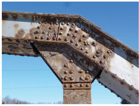
Detail of rivetted connection on metal truss [UMcA February 2015].
