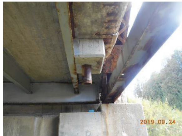
Image 14: View of the superstructure's underside, note drainage pipe
