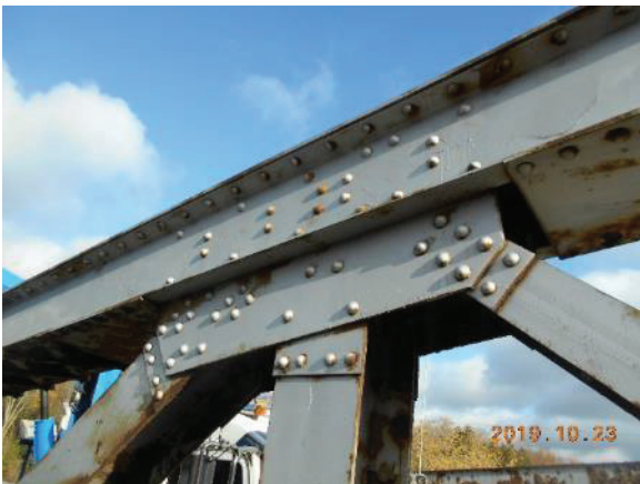
Image 9: Detail of the rivets connecting truss members
