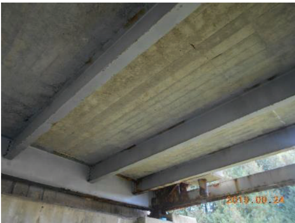
Image 13: Detail of concrete soffit, floor beam and stringer
