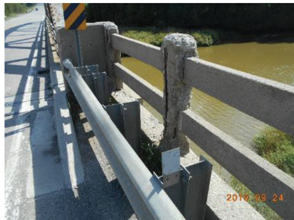
Image 16: Detailed view of concrete railings, note exposed rebar
