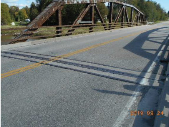
Image 17: Detail of west bridge joint and asphalt wearing surface
