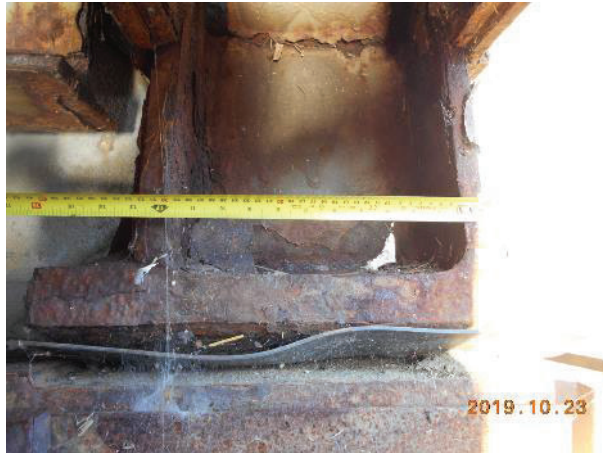
Image 19: Detail of support bearing indicating full depth section loss
