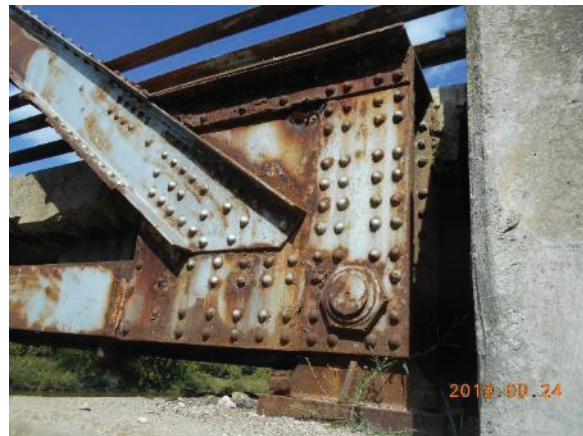
Image 10: Detail of the gusset connection
