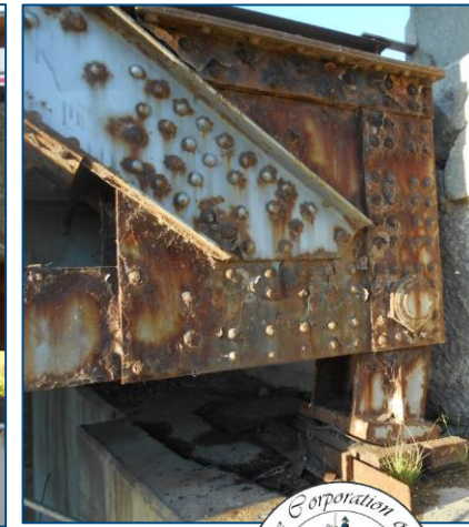
Corrosion and Rust Jacking at Gusset Connections
