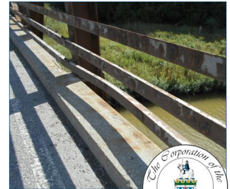
Damaged & Substandard Barrier
