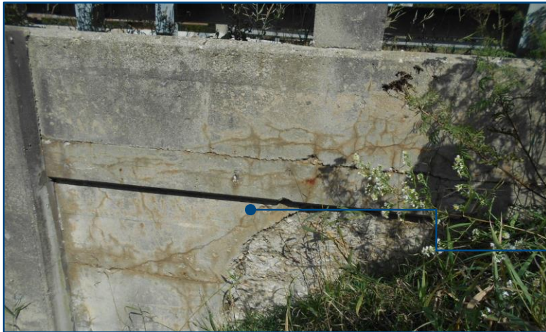
South East Wingwall
