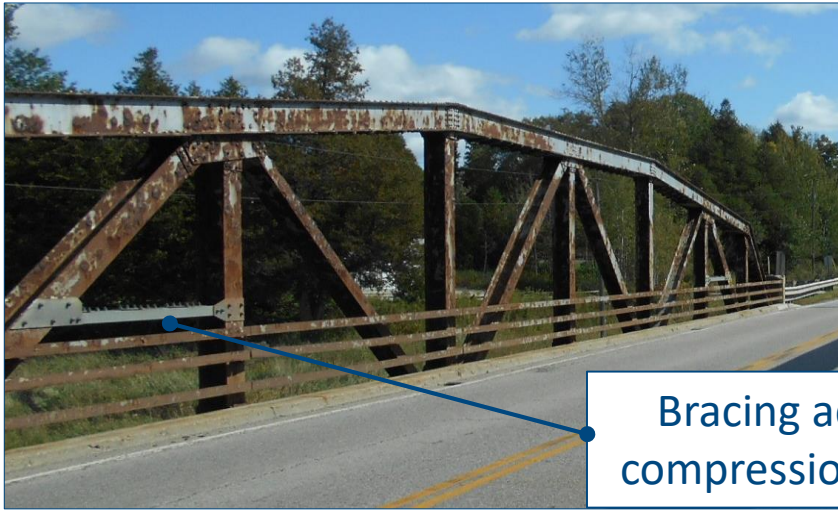
South Traffic Barrier
