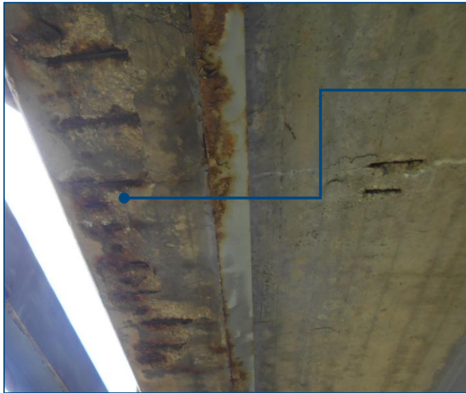
Exterior Deck Soffit
