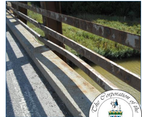
Damaged & Substandard Barrier
