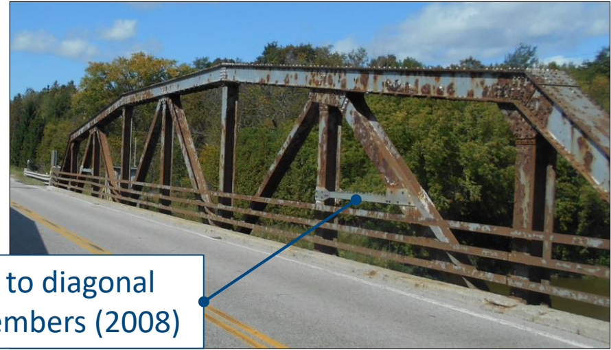
North Traffic Barrier
