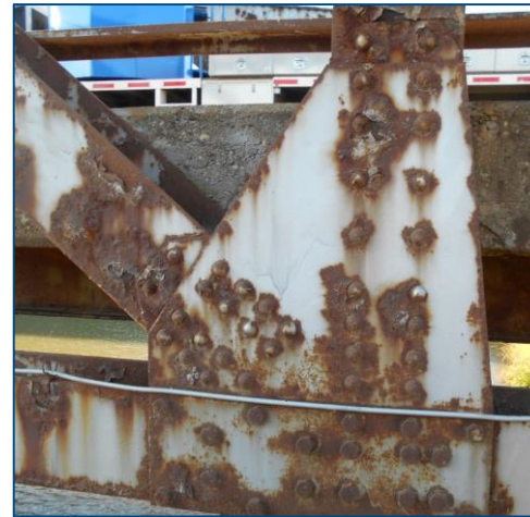
Corrosion and Rust Jacking at Gusset Connections
