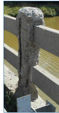
Damaged & Substandard Barrier
