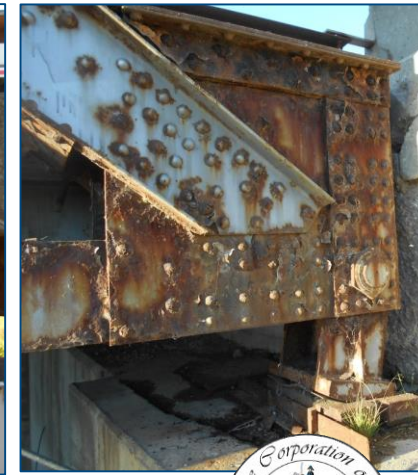
Corrosion and Rust Jacking at Gusset Connections
