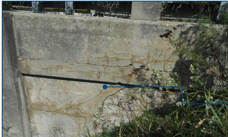
South East Wingwall
