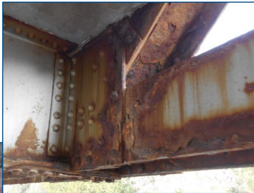
Corrosion and Rust Jacking at Gusset Connections
