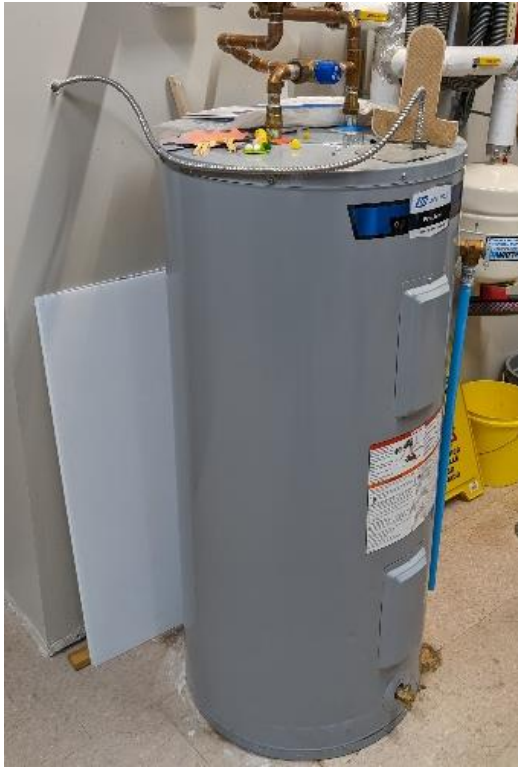
Figure 9: Electric water heater at Aboyne Library (right) and Drayton Library (left).
