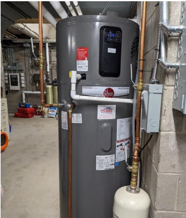
Figure 10: Heat Pump Water Heater-Court House (left) and Fergus Library (right).
