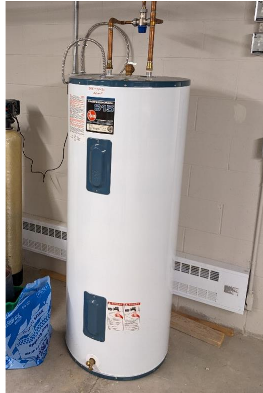
Figure 9: Electric water heater at Aboyne Library (right) and Drayton Library (left).
