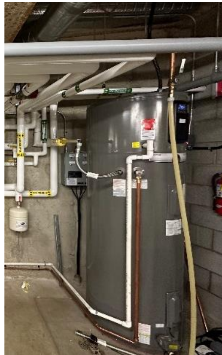
Figure 10: Heat Pump Water Heater-Court House (left) and Fergus Library (right).
