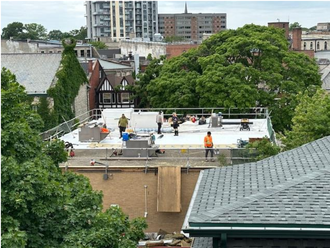
Figure 6: Roof Replacement at 21 Douglas St. 2024
