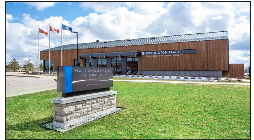
Wellington Place Child Care facility, which is currently undergoing an addition to create new childcare spaces.
