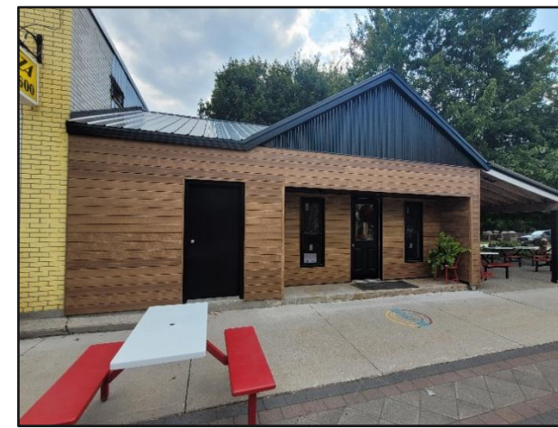
Façade improvement project, 29 Elora St in Clifford – new home of the Minto Mind Space
