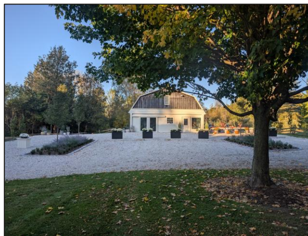
Completed renovations to Fardoire in Mapleton
