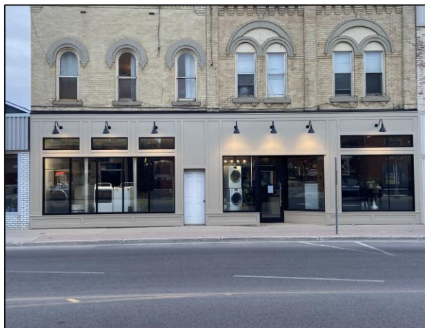
Façade improvements made to MacDonal Home Appliances Inc. in Wellington North
